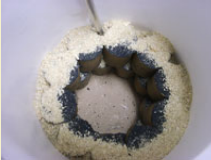
Figure 15: Tamping sawdust around gaps behind crossettes.
