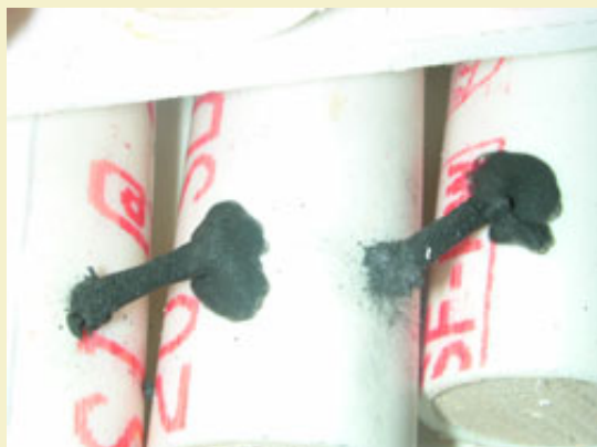
Figure 16: Painting prime slurry over holes that receive fire.
