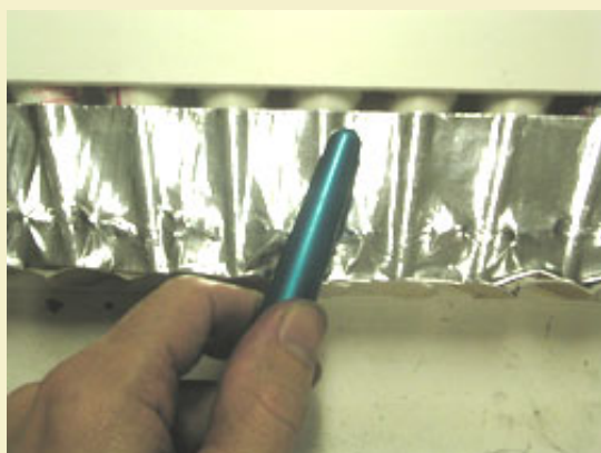
Figure 17: Making sure all air gaps under
