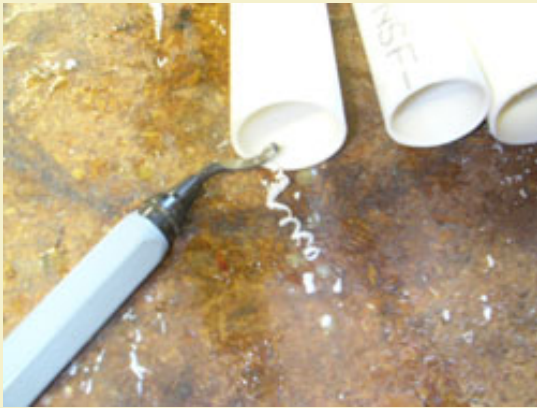
Figure 5: Using a deburring tool to trim the rough edges inside the tubes.
