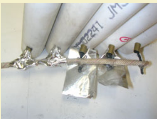
Figure 19: Protecting bare match joints with
