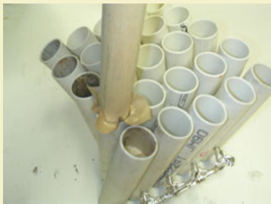
Figure 22: Pushing in paper sheets to form fire protection plugs.
