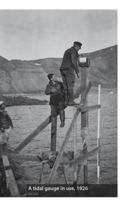
in the sand. A technological leap came in the 1800s with **wells** that used floating gauges to factor out the effects of waves. Similar techniques are still used at many coastal stations, though they've been joined lately by far more precise methods. Modern gauges measure the time it takes sound waves to bounce off the water's surface and back, converting that into distance and then to sealevel height.
