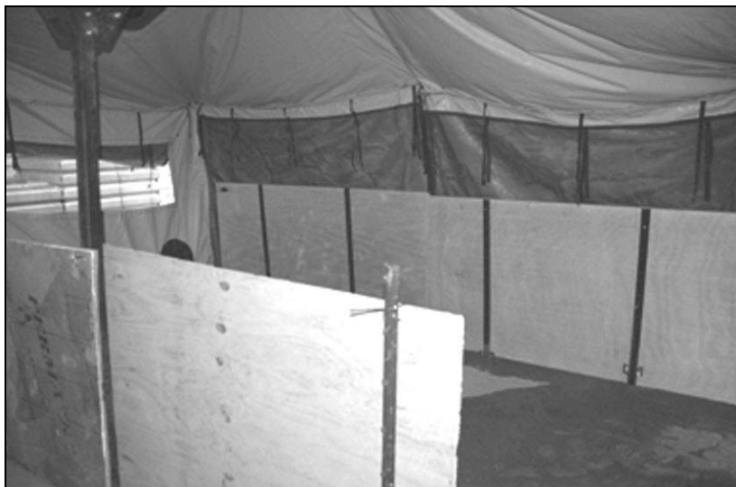
Figure 14-8. E-glass and U-picket walls used for low height protection
