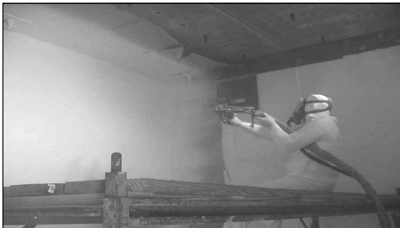
Figure 19-6. Spray-on polymer retrofit system
