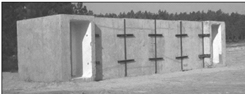
Figure 20-2. Shielded entrance concrete bunker (shown without soil cover). Steel straps connect the bunker modules together.
