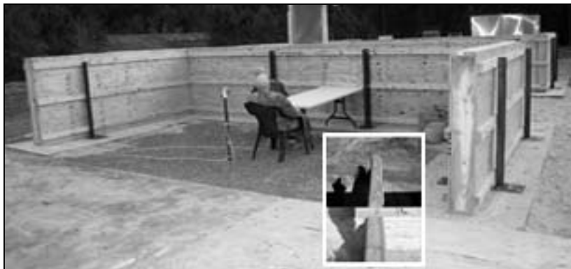
Figure 15-4. Wooden Partition Wall (Inset: Corner Joint Detail)
