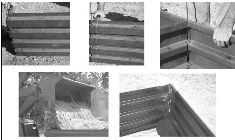
Figure D-11. Metal container infill procedure (clockwise from top left: assemble end and side panels; add cross panels; add brace panels; add poly film and wire mesh; add infill material)
