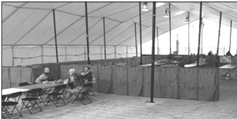
Figure 15-6. Soil-filled container walls used for compartmentalization
