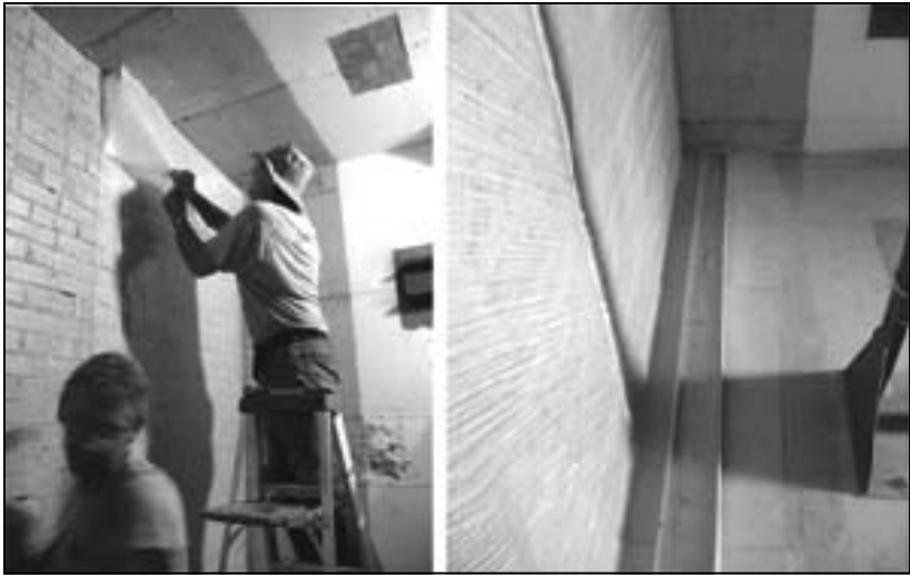
Figure 19-3. Pressure Sensitive Adhesive Retrofit (Left: application to brick wall; Right: anchoring floor to slab)
