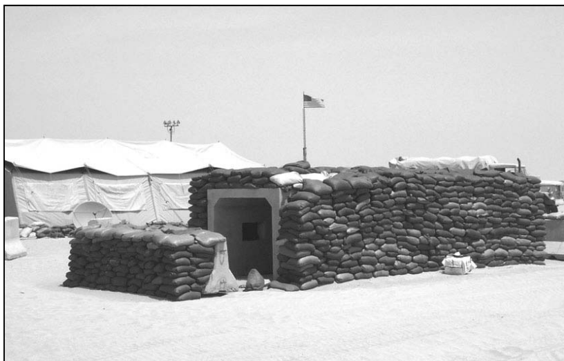
Figure 20-1. Improvised bunker using concrete culvert sections. Sandbags provide increased fragmentation protection from near-miss weapons.
