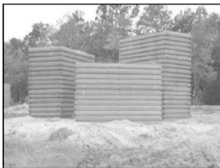
Figure 12-17. Typical Metal Container Revetment Barrier
