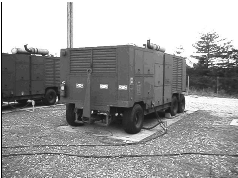
Figure 7-4. Typical Prime Power Generator
