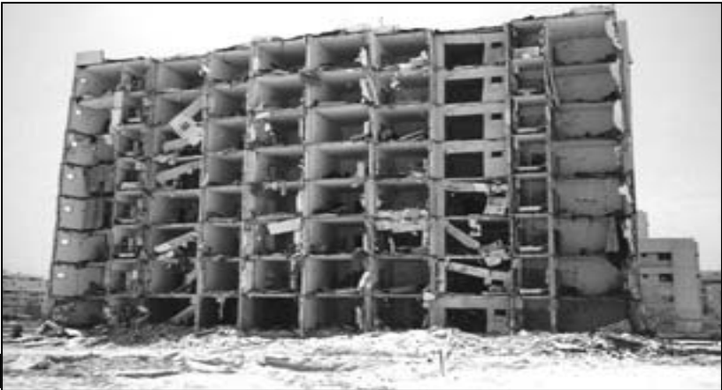
Figure 11-7. Building damage resulting from the 1996 Khobar Towers attack
