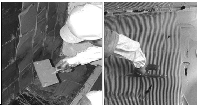
Figure 19-7. Trowel-on polymer retrofit system
