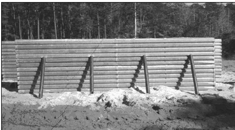
Figure 14-5. Bracing metal revetment walls for near-miss 122-mm rocket threat. Bracing here is provided by steel pipe; 4 x 4 timbers can also be used.
