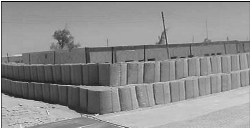
Figure C-2. Example of a perimeter wall using soil-filled wire and fabric containers
