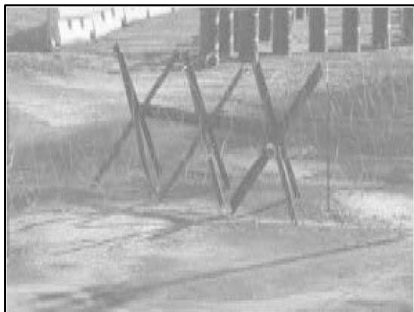
Figure 12-14. Typical Cabled Steel Hedgehog Obstacle
