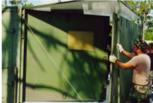
Figure 4.7. Positioning Swing-out Sidewalls.
