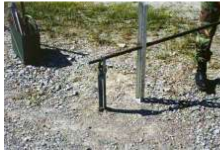
Figure 6.35. Pulling Shear Stakes.
