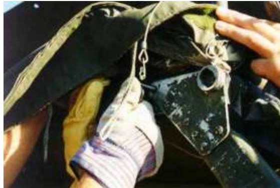
Figure 3.32. Securing Purlin Flaps.
