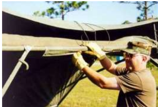
Figure 3.32. Securing Purlin Flaps.
