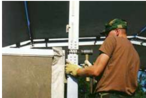
Figure 6.26. L2/LU-2 Column Connection.
