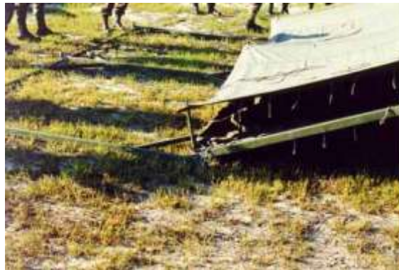
Figure 3.27. Tent Fly in Place over Eave Extenders.
