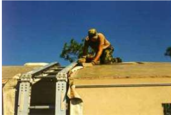
Figure 6.23. Ridge Flashing Installation.
