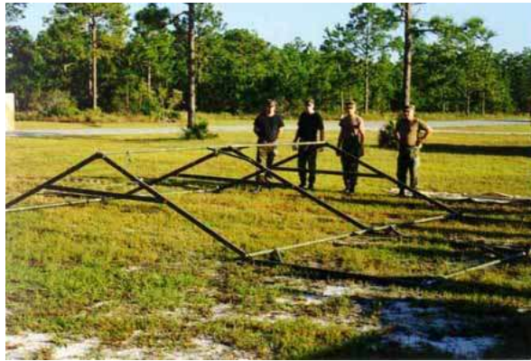
Figure 3.17. Assembled TEMPER Tent Frame.
