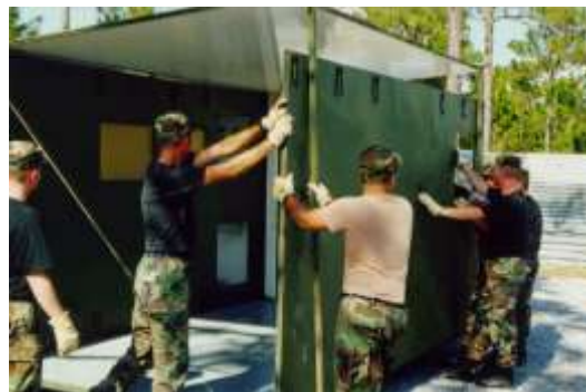
Figure 4.6. Raising End Wall.
