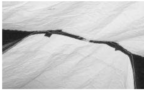
Figure 2.30. Second Liner Attached to Face of First Liner.
