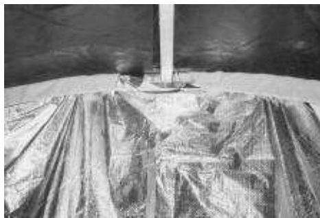
Figure 2.31. Liner Attached to End Panel.
