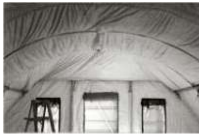
Figure 2.24. Interior Liner Panel Installed.
