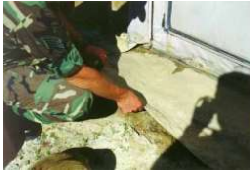
Figure 6.34. Installation of Ground Skirt Flashing.
