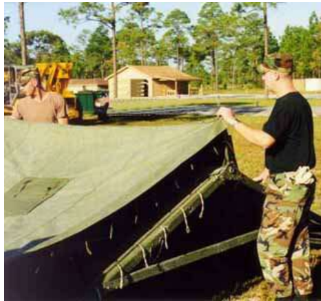
Figure 3.25. Placement of Tent Fly Over Ridge Extenders.
