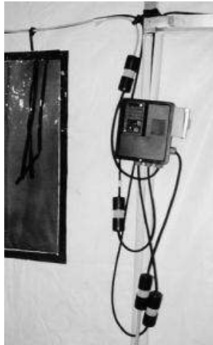
Figure 2.33. Plastic Distribution Box Installed.
