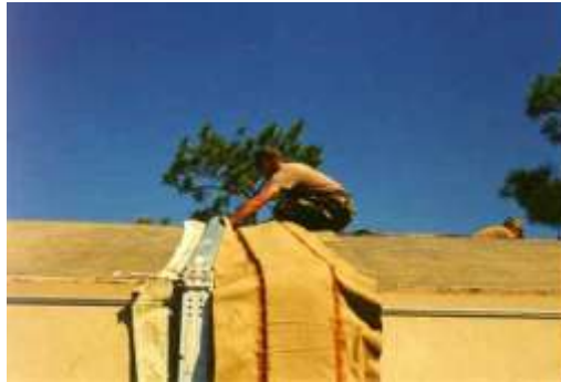
Figure 6.33. Arch Counterflashing Attachment.
