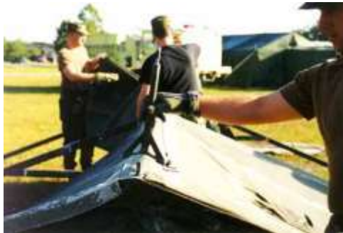
Figure 3.23. Installation of Ridge Extenders.
