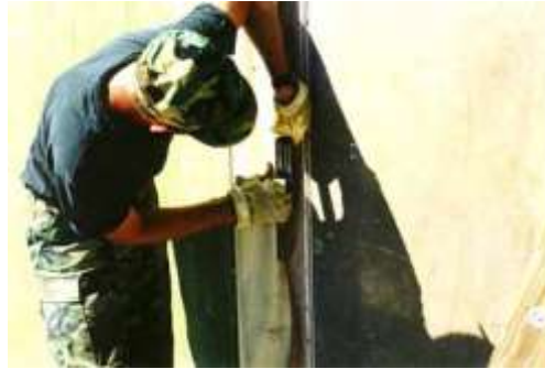
Figure 6.30. Door Flashing Attachment.
