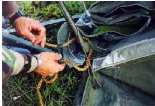
Figure 3.29. Attachment of Guy Ropes to Eave and Ridge Extenders.
