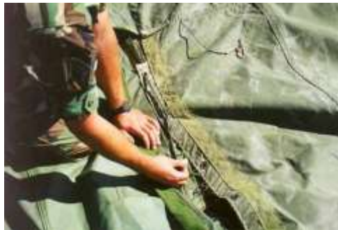
Figure 3.24. Lacing of Tent Fly.
