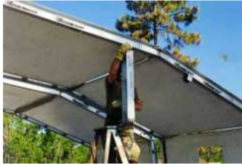
Figure 6.24. Column Attachment to Arch Beam.
