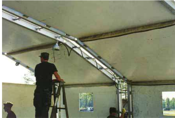
Figure 6.21. Lighting Fixture Cable Run.
