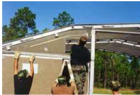
Figure 6.27. Upper Panel Section Placement.
