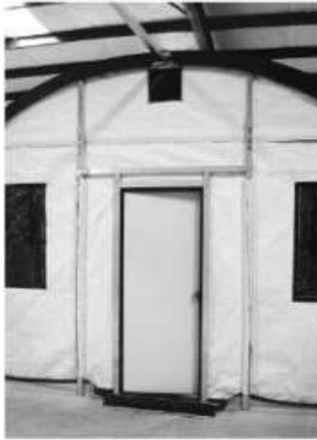
Figure 2.16. Hard Door End Panel Installed.
