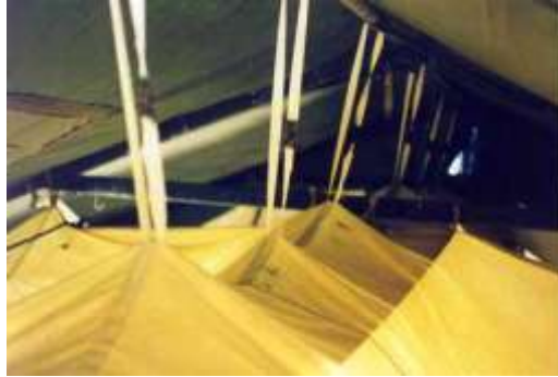
Figure 3.37. Overhead Liner Connections.
