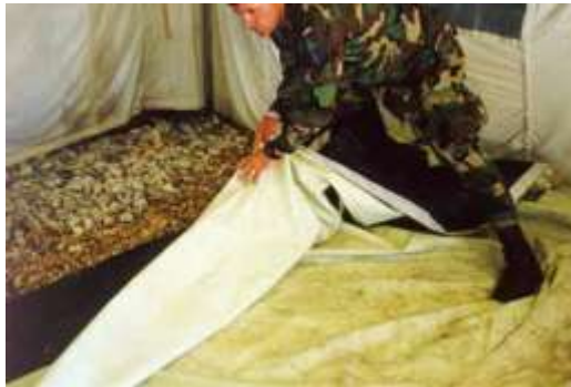
Figure 3.34. Flooring Section Installation.
