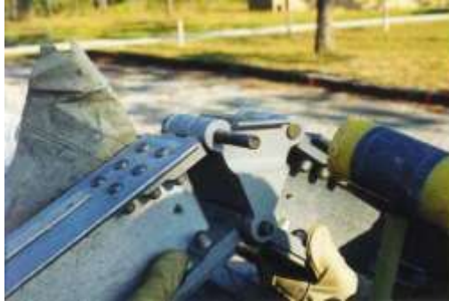
Figure 6.10. Beam-to-Beam Pin Connection.
