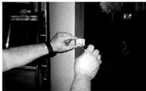
Figure 2.17. Removal of Door Bracket.
