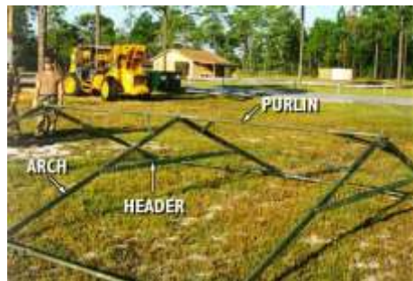
Figure 3.3. TEMPER Tent Frame Components.
