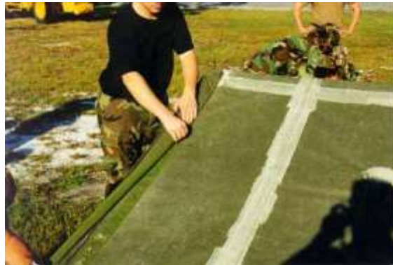
Figure 3.20. Closing of Hook and Pile Fastener Weather Flap.
