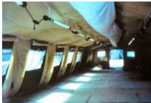
Figure 3.5. Installed Liner with Plenum and Lighting.
