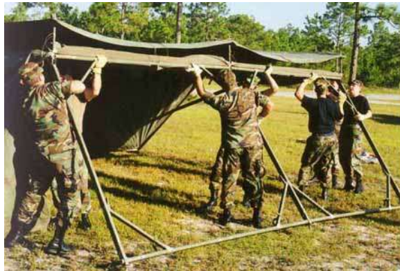
Figure 3.30. Raising Tent Frame Assembly.
