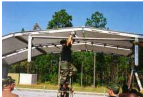
Figure 6.25. Installation of Header.
