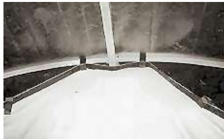
Figure 2.27. Attaching Center Hook and Loop Fasteners on Center Arch.
