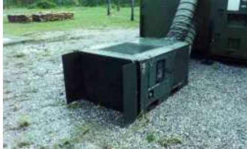
Figure 4.13. Environmental Control Unit Installation.
