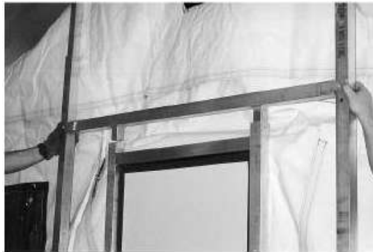
Figure 2.15. Sliding Header Stubs into Top of Door Frame.
