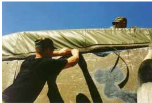
Figure 6.31. Attaching End Wall Flashing to End Wall Panels.
