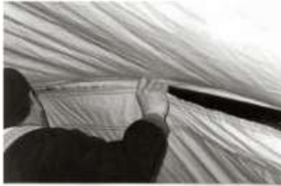
Figure 2.24. Interior Liner Panel Installed.
