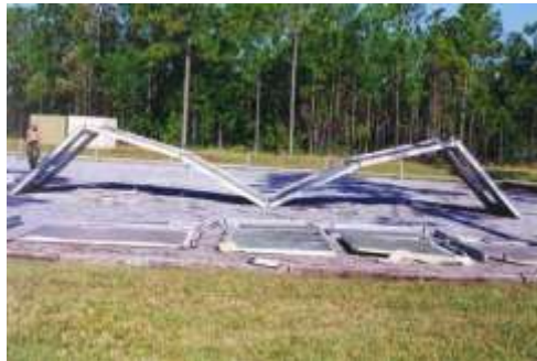
Figure 6.13. Placement of Panel Sections Prior to Erection.
