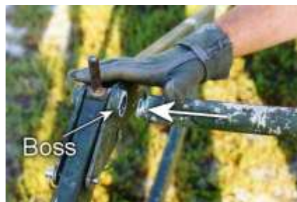
Figure 3.14. Purlin-to-Arch Connection.
