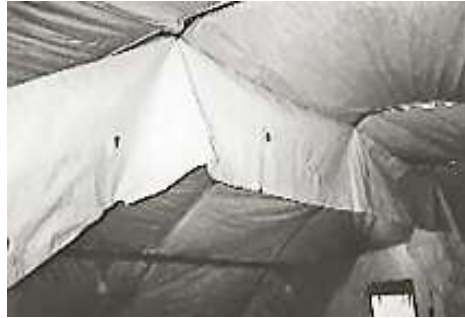
Figure 2.37. Plenum Attachment to ECU Supply Duct.
