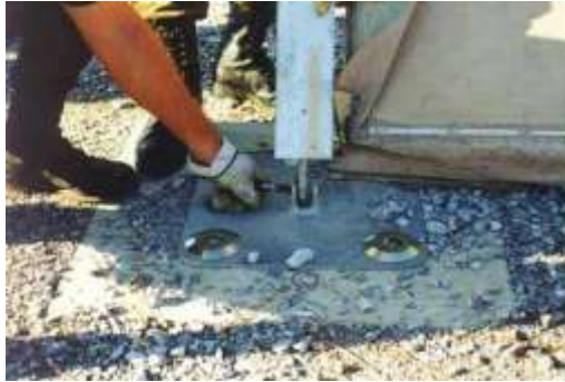
Figure 6.11. Pinning of Panel to Basepads.
