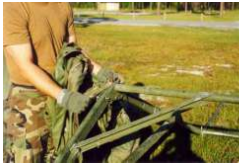
Figure 3.22. Placement of End Wall Peak Grommet.
