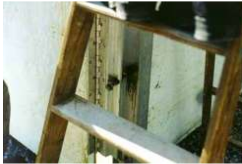
Figure 6.29. Door Hinge Mounting Bolts and Column Mounting Inserts.
