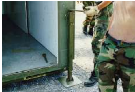
Figure 4.2. Jack Installed at Corner of Center Section.
