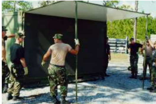
Figure 4.4. Raising Roof Panel.
