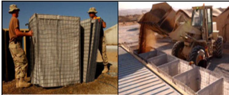
Figure 2.23. Wire Mesh Containers Being Expanded and Filled On-Site.
