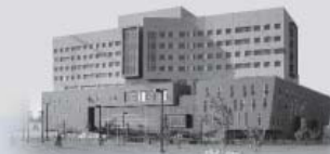
Bomb Shelters, Buildings, Critical Infrastructure
