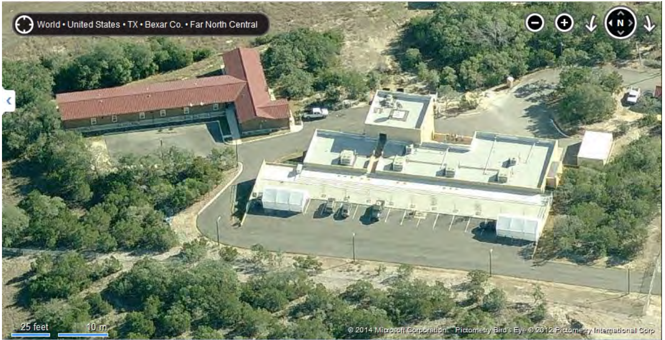
New construction in outer cantonment.
