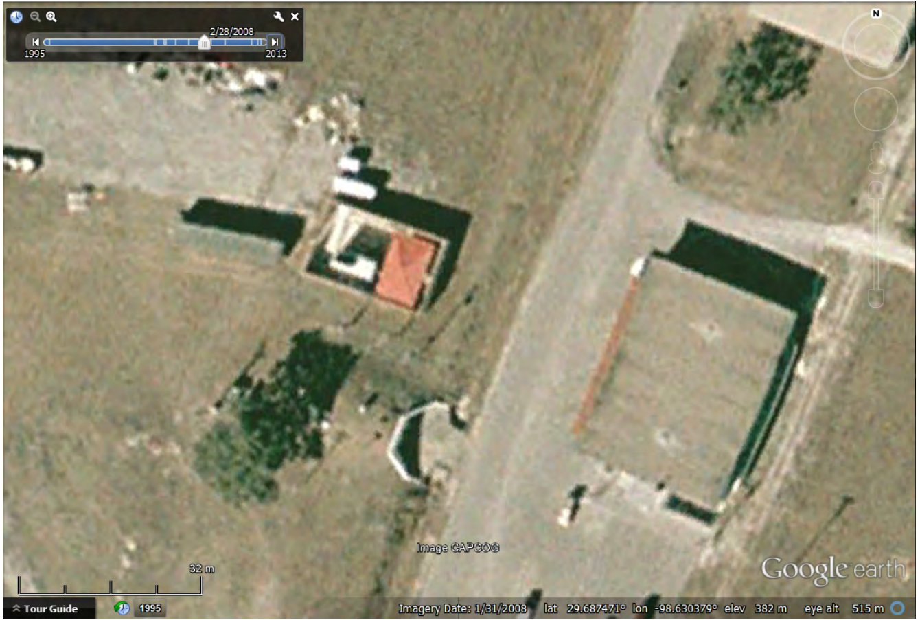
One generator set, 2008-01-31
