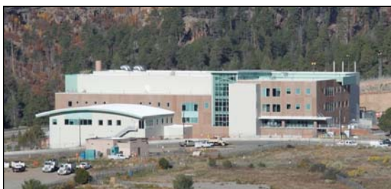
Figure 5. Radiological Laboratory/ Utility/Office Building
