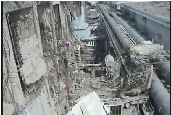
T-Hawk image -seashore-side of the reactor building.
