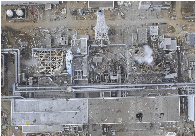
March 20, 2011, Damaged Unit 4 (left) and damaged unit 3 (right) from the Air Photo Service UAV.
