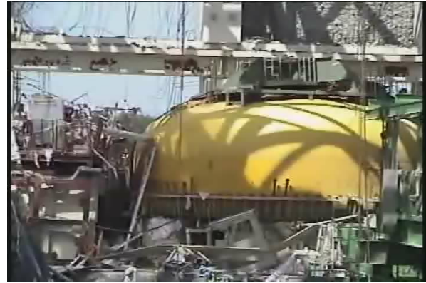
T-Hawk image of operation floor of a reactor building
