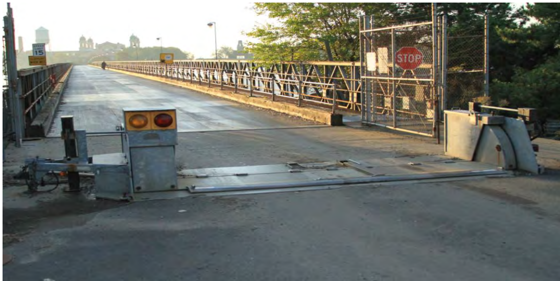
Photo No. 1 Ellis Island Bridge Vehicle Barrier
