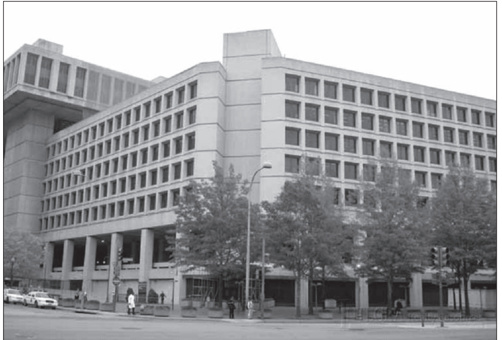
Figure 1: J. Edgar Hoover Building Facing Pennsylvania Avenue and 10th Street
