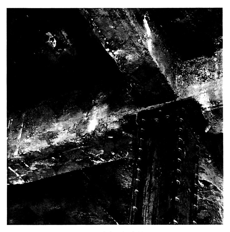
GOOD EXAMPLE OF EXISTING CONCRETE ENCASEMENT FINISH: MODERATE IMPERFECTIONS AND TEXTURE, WITH DEFINED BEAM EDGES AND STRUCTURAL COVERAGE OF ENCASED STEEL BEAMS
