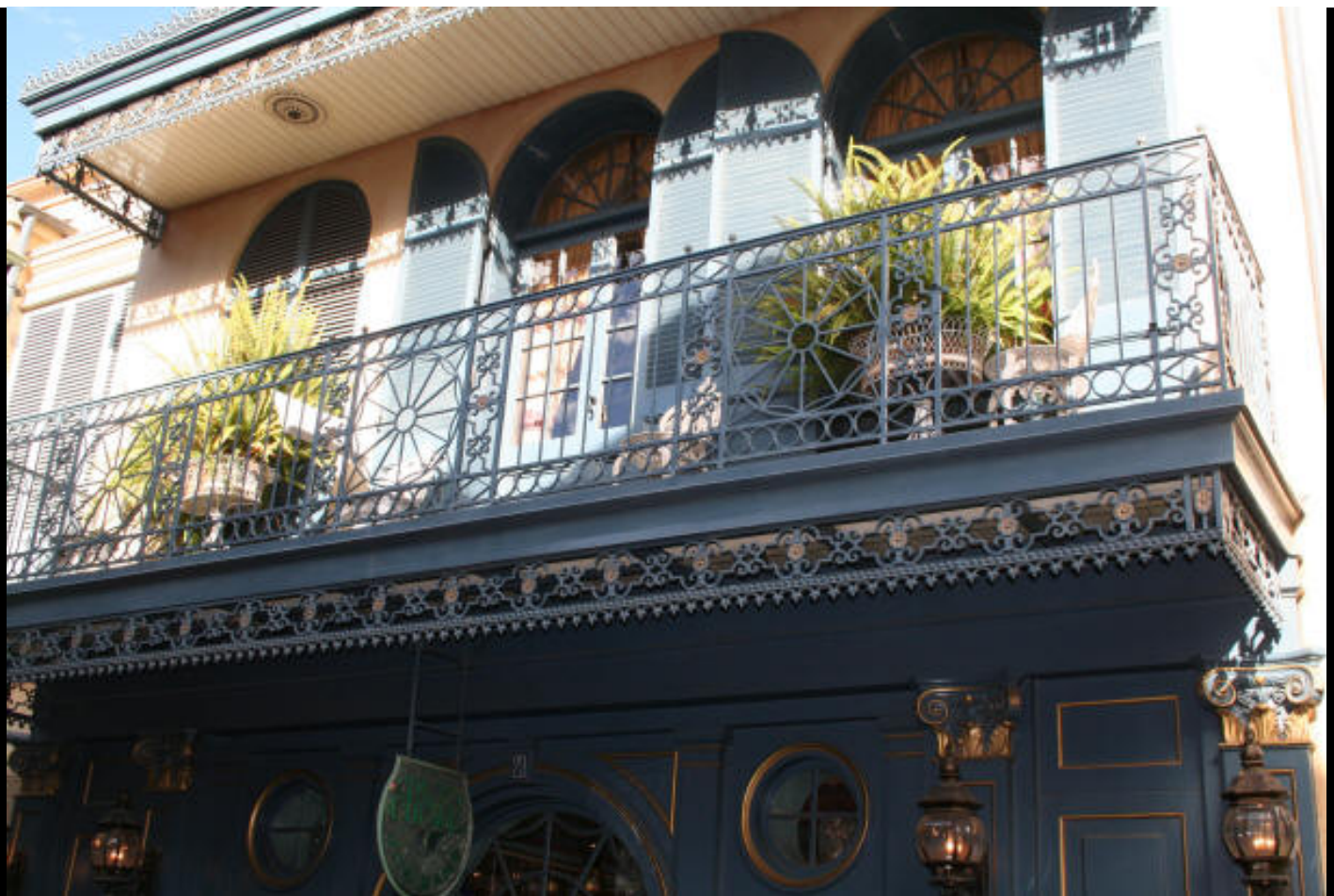
Here we display the West balcony of the Lounge Alley.
