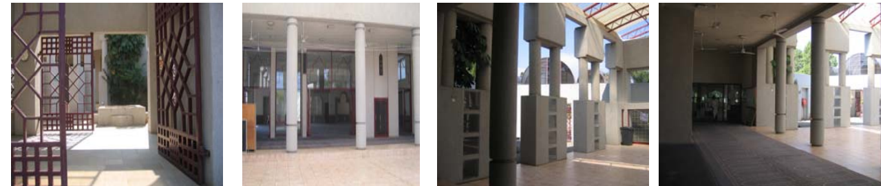
(Fig.'s 7-10. Local studies). Friday Mosque, Brits, 1998 – uses repetition in material, colour and architectural elements to create the rhythm in the absence of the arched colonnades.
