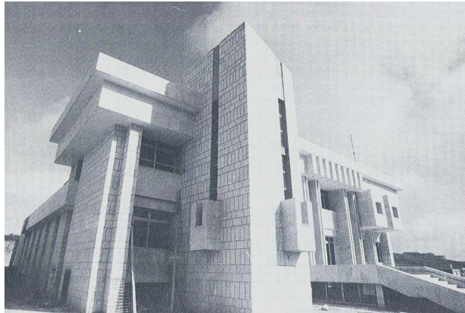
(Fig. 114. Global study). Press and publication building, Amman, Jordan (Picture from Lari: 1990, p.143).
