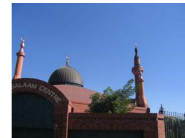
Adjacent: (Fig.'s 29-30. Mosque analysis). Dome placed at centre the of the Dar-as-Salaam Mosque, to portray an Islamic eminence.
