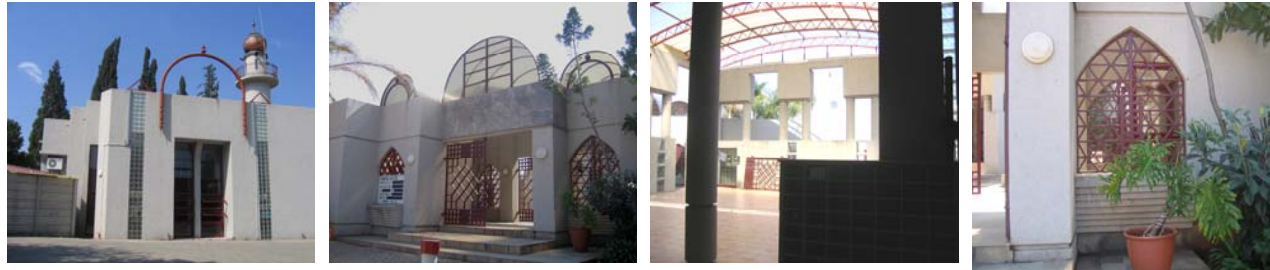
Rusty red aluminium arch attached to wall with linear elements (Fig.'s 11-14. Local studies). Arched skylights placed above linear main entrance (Fig.'s 11-14. Local studies). Arched semi-permeable roof attached to linear columns (Fig.'s 11-14. Local studies). Pointed arched window within linear setting (Fig.'s 11-14. Local studies). Friday Mosque, Brits, 1998 – uses arches in an innovative manner, to create a theme of the past within a new context.
