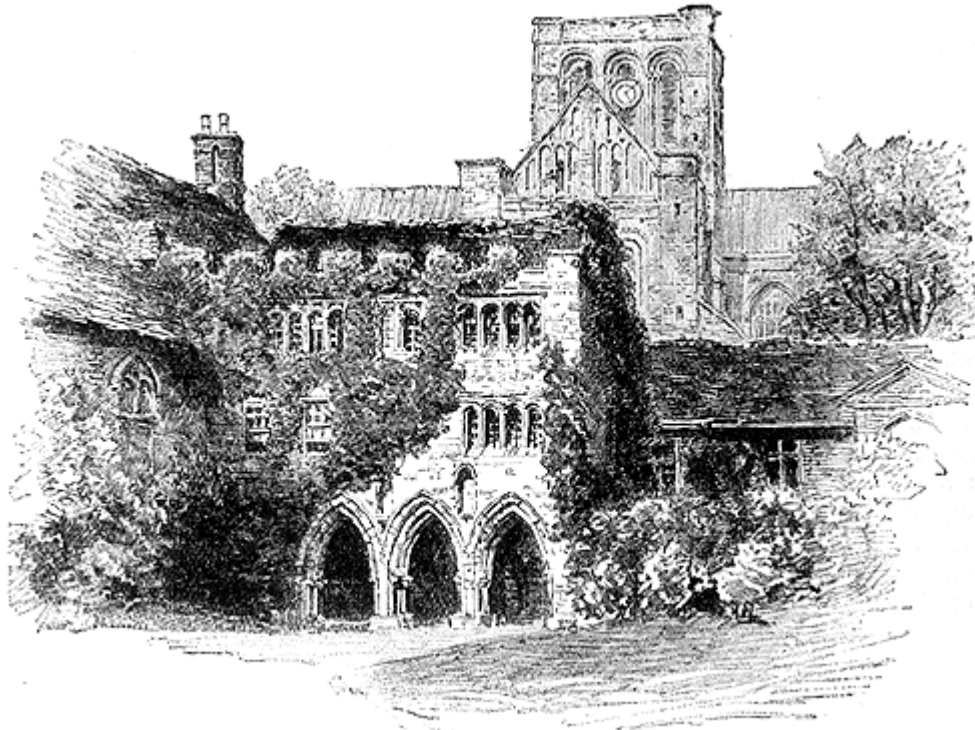
VIEW OF THE DEANERY AND CATHEDRAL AT WINCHESTER.
