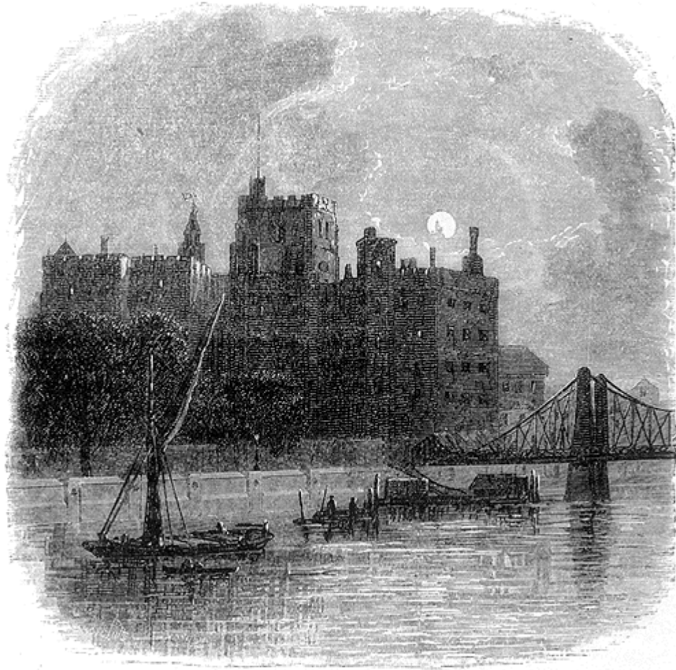
VIEW OF LAMBETH PALACE.
