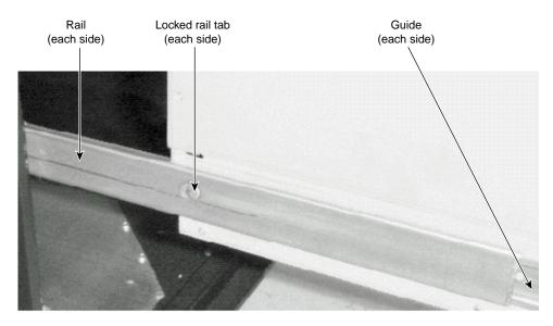
Figure 1-8 Rail on Rail Guide
