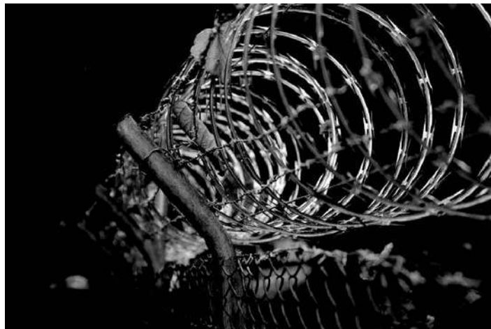
Figure 9.6 Coiled razor wire on chain link fencing looks intimidating but is easily defeated.
