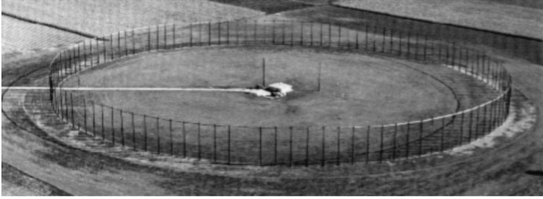
Figure 10.1 Wullenweber array. (Source: [1], © University of Illinois. Reprinted with permission.)
