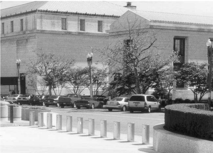
FIGURE 9.4 Raised stainless steel bollards protect access to the U.S. Department of State headquarters. (Courtesy of Delta Scientific, Inc.)
