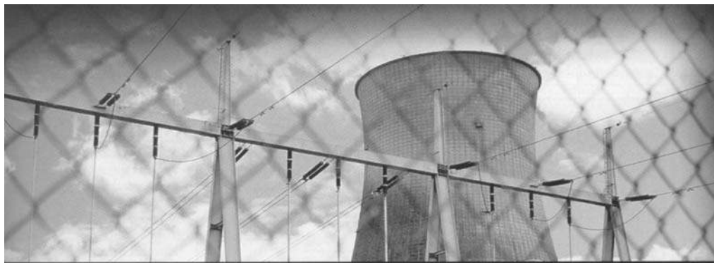
FIGURE 1.2 A nuclear power facility.
