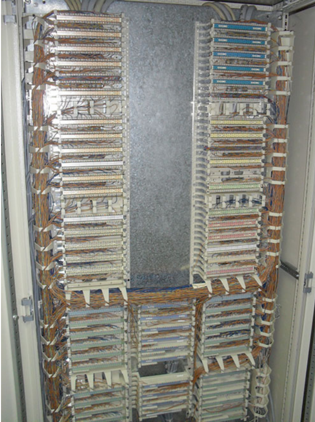
Fig. 4.6 Large distribution frame (>1000 connections)
