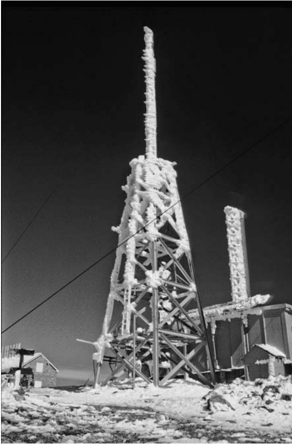
Figure 9.8. Severe riming on a tower at the summit of Mt Washington, New Hampshire (1917 m / 6288 ft) in May 1991. The small building on the left was the original Mt Washington Observatory, which held the record for the world's highest measured wind speed until 1996. (Photograph by the author)
