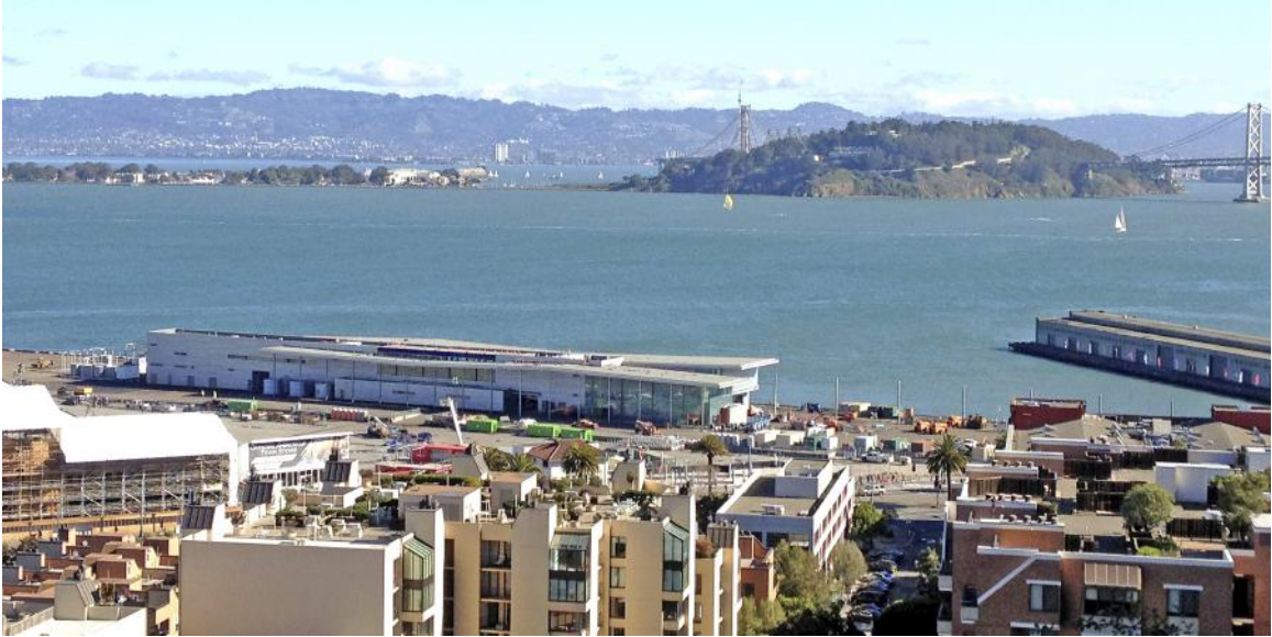
Figure 1.12 Designed as a welcoming gateway to the city, as well as an active hub for large cruise ships, Pier 27 Terminal is built on the impervious surface of a large San Francisco pier. Rainwater harvesting was employed as a means to provide flushing for toilets in the building designed by KMD Architects with Pfau Long Architecture. ( KMD ARCHITECTS + PLA, & PFAU LONG ARCHITECTURE, a Joint Venture )
