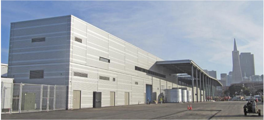
Figure 1.13 Three aboveground rainwater collection tanks are sized to meet both the monthly demand for toilet flushing and for irrigation at Pier 27. (KMD ARCHITECTS & PFAU LONG ARCHITECTURE, a Joint Venture)
