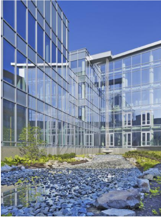
Figure 3.4 Rainwater waterfall at the NOAA Center for Weather & Climate Protection, College Park, Maryland, USA. (Alan Karchmer, courtesy of HOK)
