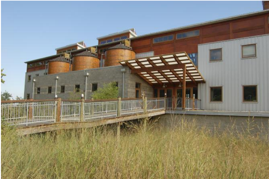
Figure 1.20 The 2001 Philip Merrill Environmental Center, designed by SmithGroup for the Chesapeake Bay Foundation, was the first Platinum LEED® building. This project demonstrates that a design that includes a number of sustainable strategies including rainwater harvesting can save energy and water resources. (Photo courtesy of the Chesapeake Bay Foundation/www.cbf.org)
