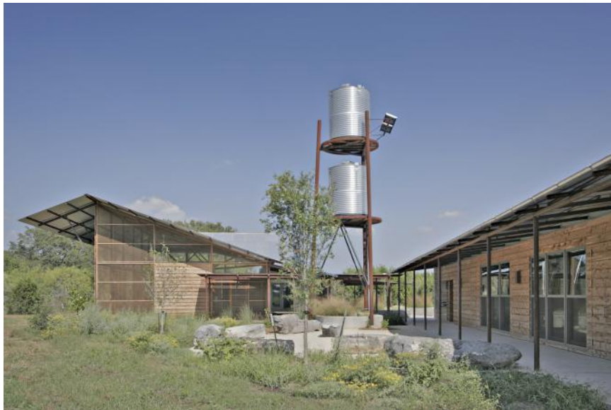
Figure 2.14 The high-use, low-maintenance, and economical structures at the Government Canyon Visitor Center reinforce the mission of the client. ( Chris Cooper )
