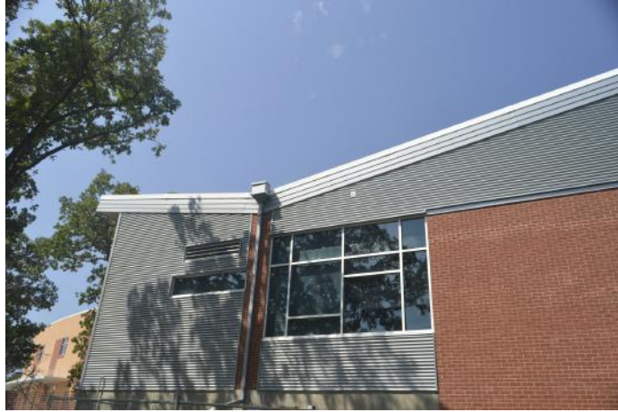
Figure 4.6 A butterfly roof in Denton, Texas, offers aesthetics and a convenient catchment point for rainwater. ( Eddie Van Giesen )
