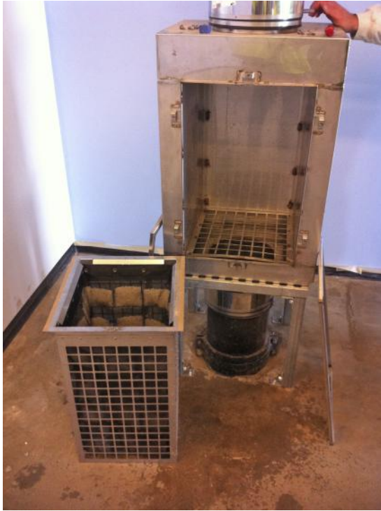
Figure 4.15 Large capacity downspout filter with built-in overflow. This filter is installed vertically and must be accessible for ease of cleaning as water cascades over the screen. (Eddie Van Giesen)
