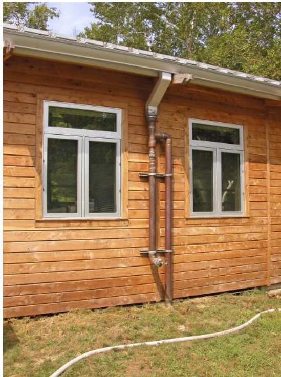
Figure 5.19 Tyson Living Learning Center downspouts with rain diverter. (Ralph Bicknese, Hellmuth + Bicknese Architects)
