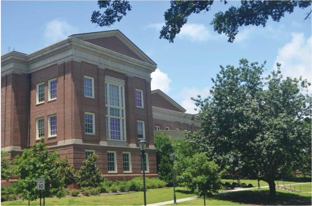
Figure C.3 The Paul Coverdell Research Center at the University of Georgia in Athens, Georgia, uses rainwater for toilet flushing and cooling tower makeup water. ( Viviane Van Giesen )
