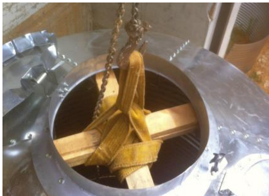
Figure 4.23 Corrugated tank with access opening is attached to the top section of the tank. (Eddie Van Giesen)
