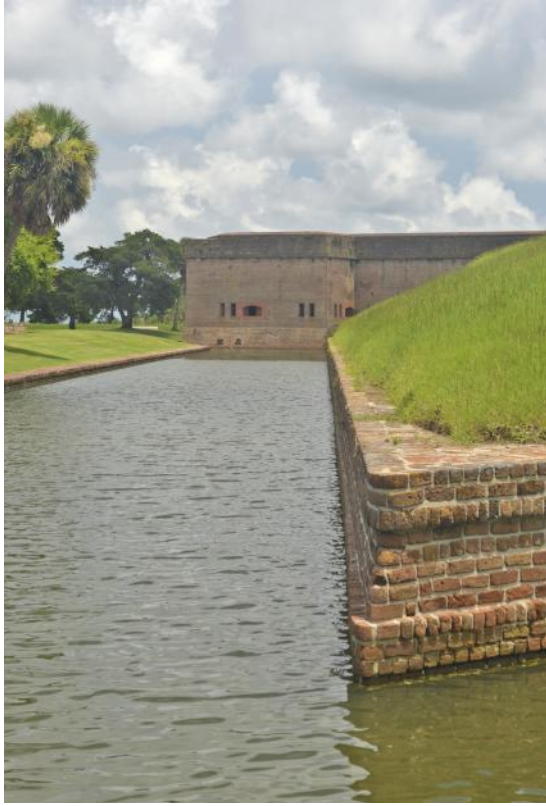
Figure 1.6 Fort Pulaski National Monument in Georgia provides an example of a historic rainwater collection system. Ten brick subterranean cisterns incorporated into the structure of the fort were capable of storing 200,000 gallons of fresh water. After the capture of the Fort, in 1862, Union soldiers supplemented the natural supply with a steam condenser which converted the moat's saltwater into freshwater. ( Eddie Van Giesen )
