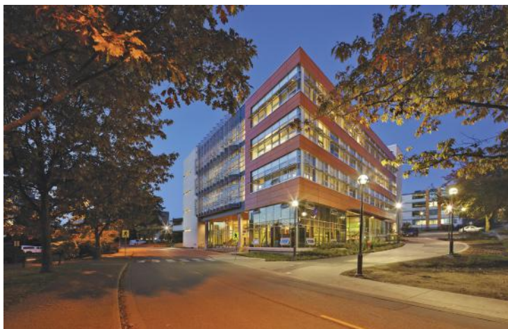
Figure 5.14 Research on sustainability designed by Perkins+Will Architects has an extensive rainwater harvesting system. ( Centre for Interactive )
