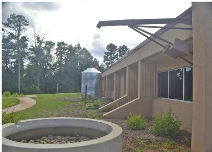
Figure 4.14 Exaggerated conveyance provides educational opportunities in a rain garden/rainwater harvesting system for the Fowler Drive Elementary School, Athens, Georgia. ( Viviane Van Giesen )
