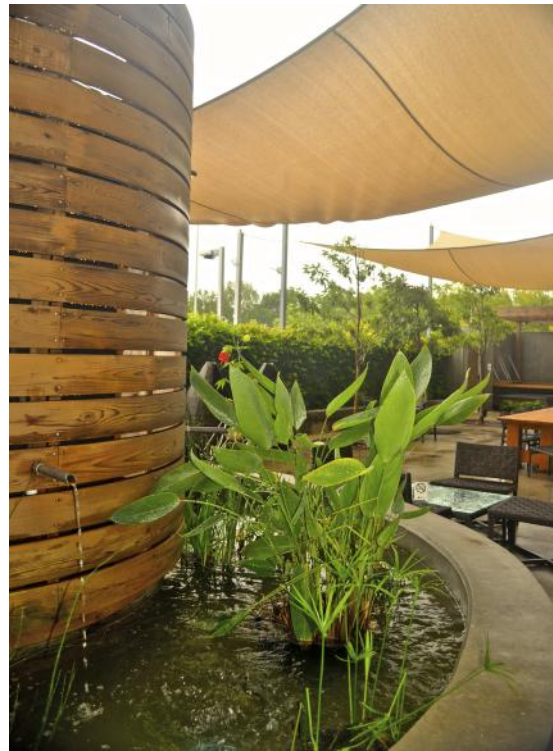
Figure 4.27 Wood cladding transforms a utilitarian plastic tank into an attractive fountain feature. (Vivian Van Giesen)
