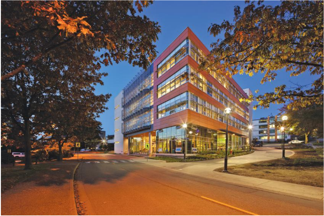
Figure C.7 Center for Interactive Research on Sustainability, designed by Perkins+Will Architects, has an extensive rainwater harvesting system. ( Martin Tessler / Courtesy: Perkins+Will )
