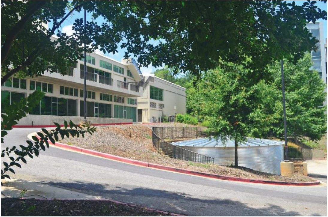
Figure C.11 An integrated system provides water for toilet flushing and cooling towers at the University of Georgia Visual Arts Building. ( Viviane Van Giesen )
