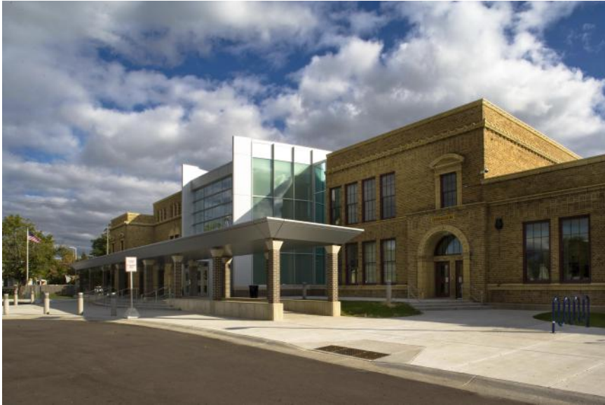
Figure 3.13 Burton Elementary and Middle School in Grand Rapids, Michigan was designed to collect rainwater to flush toilets and water closets as part of a sustainable renovation to this historic building. (Brian Kelly)
