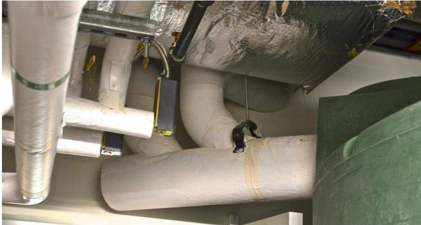
Figure 4.11 Insulated leaders from a flat roof convey water inside the building envelope to a rainwater tank. (Eddie Van Giesen)
