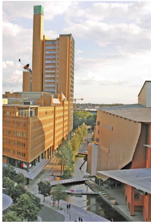
Figure 1.11 Potsdamer Platz integrates various water system designs to create a vibrant natural area in the heart of Berlin. ( Judy Leel/Atelier Dreiseitl )
