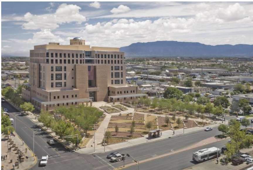
Figure 2.7 Landscape architect Rios Clementi Hale Studios collaborated with water system designer Biohabitats to meet stormwater regulations and challenges by using rainwater as part of the design methods for irrigation at Pete V. Domenici U.S. Courthouse in Albuquerque, NM. (Robert Reck)
