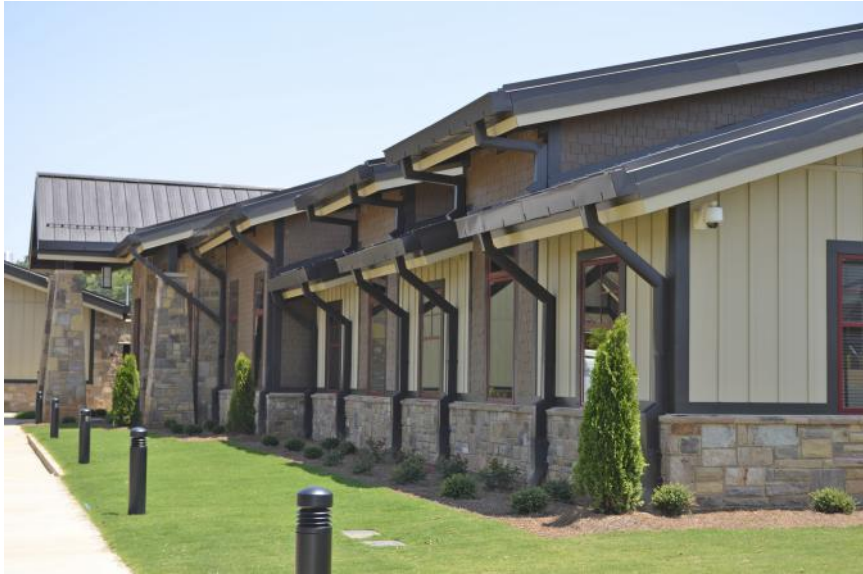
Figure 4.13 The gutters and downspouts used on this building repeat as part of balanced modules in the facade of Blue Ridge Electric Membership Cooperative, Young Harris, Georgia. With over 100 downspouts, they serve as a strong visual element in the facade of the building. ( Eddie Van Giesen )
