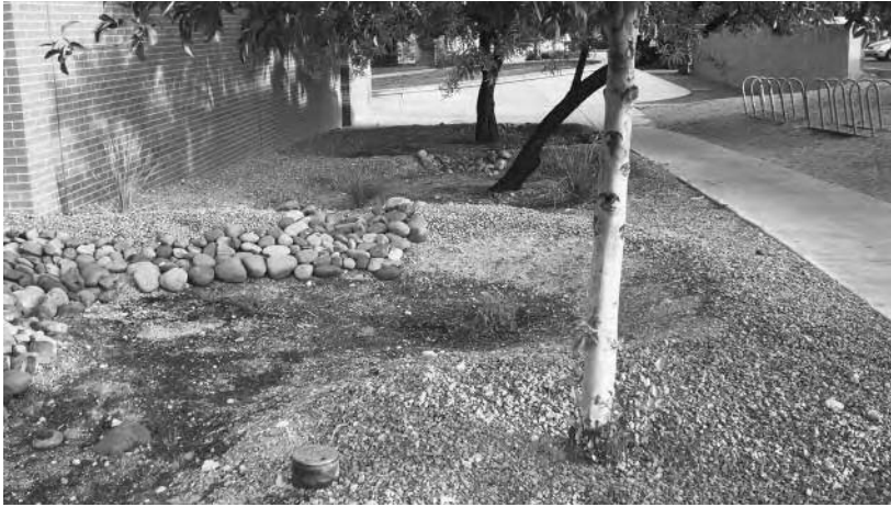
Stepped stormwater basins manage overflow from other basins fed from downspout drains
