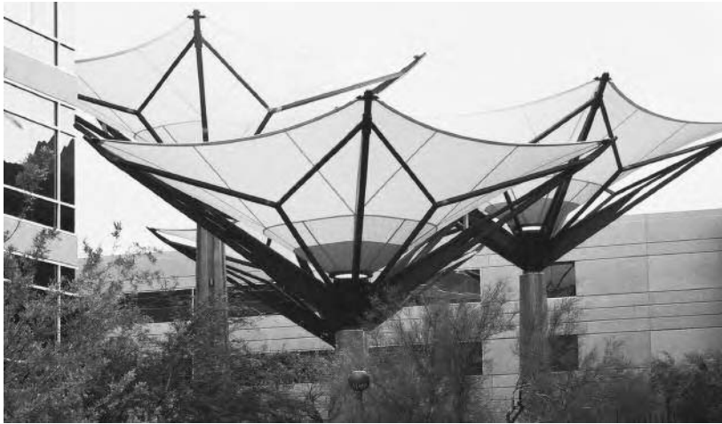
Rain-catching, shade-providing, upside-down umbrellas in a courtyard of multiple commercial office buildings
