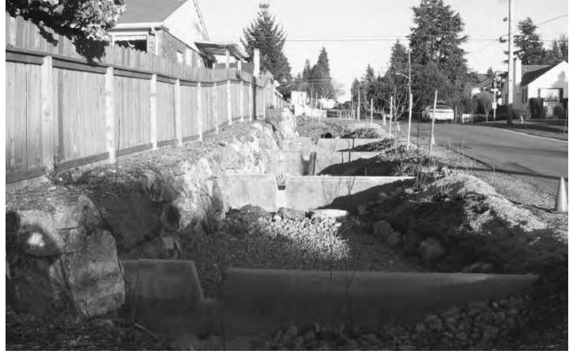
Stepped cascade rain gardens at initial completion
