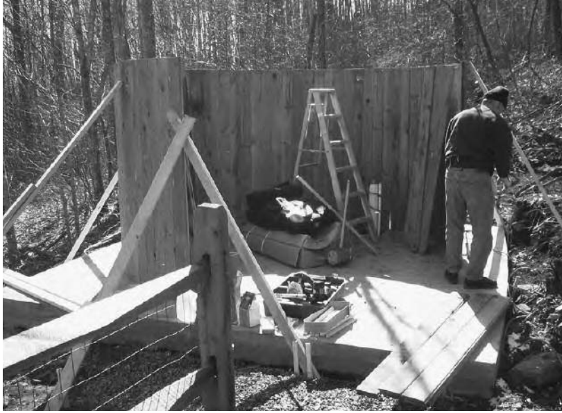
Wooden tank construction in cold climate – sides
