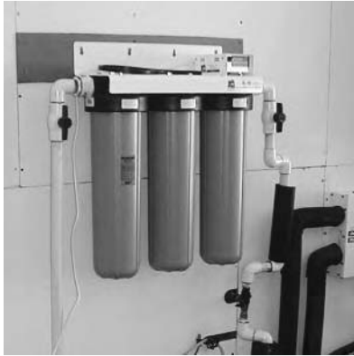
Left to right are 3 filters: a 5-micron sediment filter, a 0.5 micron carbon filter, and UV purification
