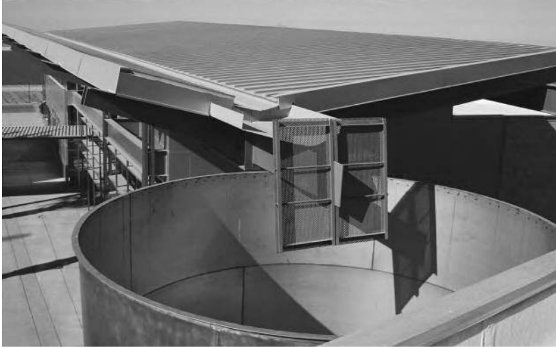
Butterfly roof gutter and splash panel to stainless steel tank
