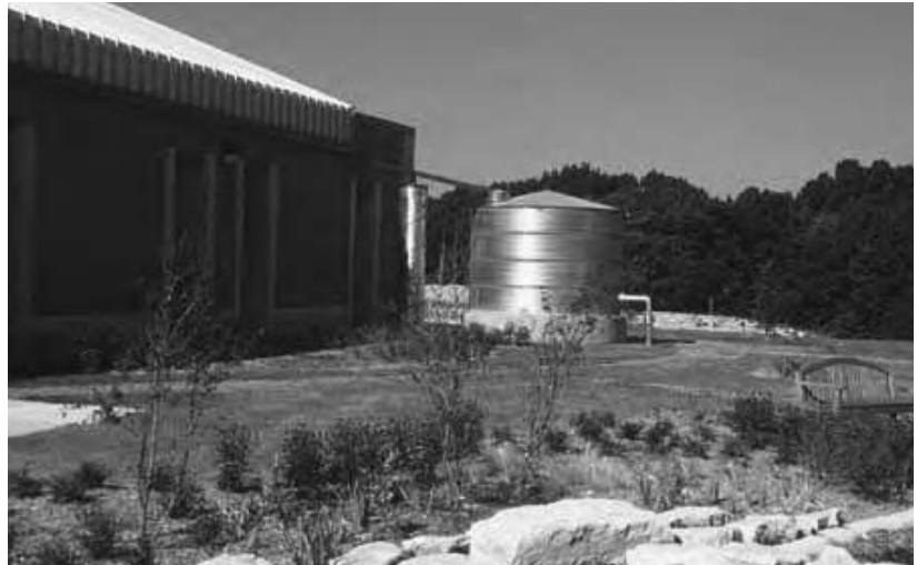
View of cistern at the back of the school from the courtyard
