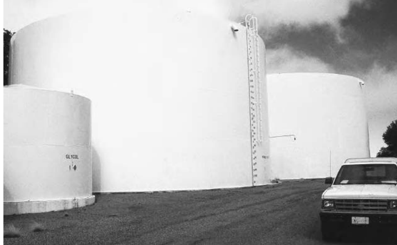
Two 500,000-gallon storage tanks
