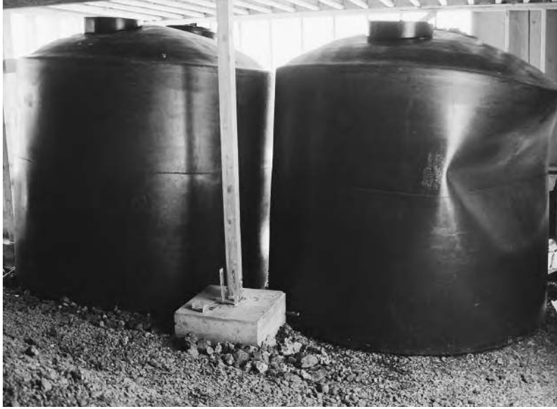
Empty tanks under a wooden deck ready for installation
