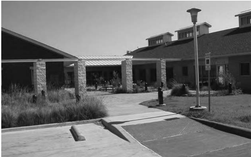
Aqueduct over entry
