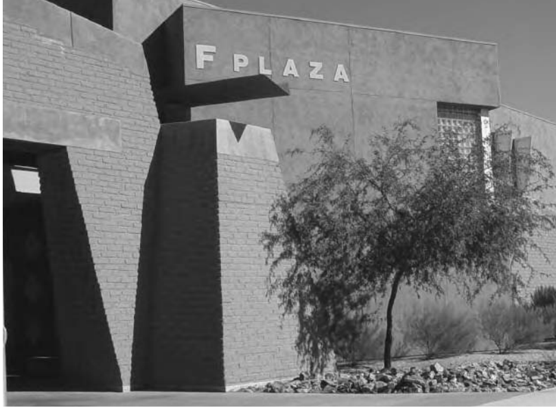
Passive rainwater harvesting: Pima Community College F Plaza gutter drops to splash pad of rocks next to a tree
