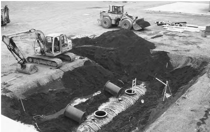
Rainwater tank installation
