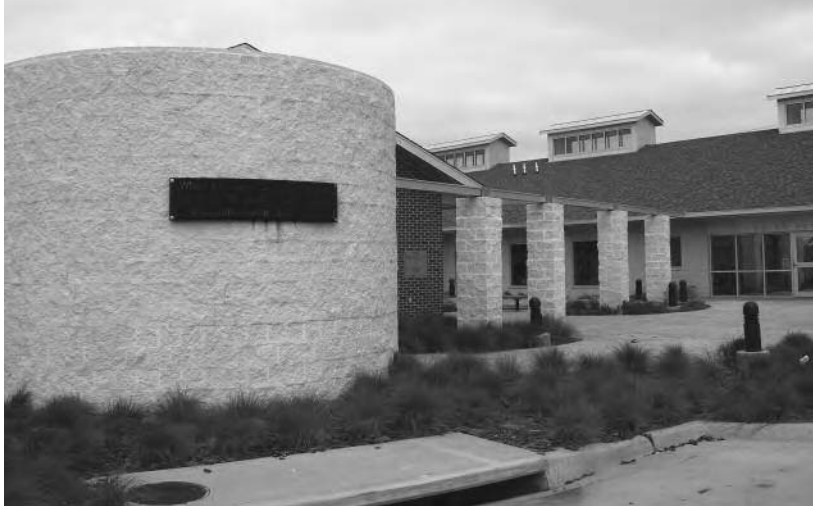
Front of the animal shelter with the entry rainwater tank
