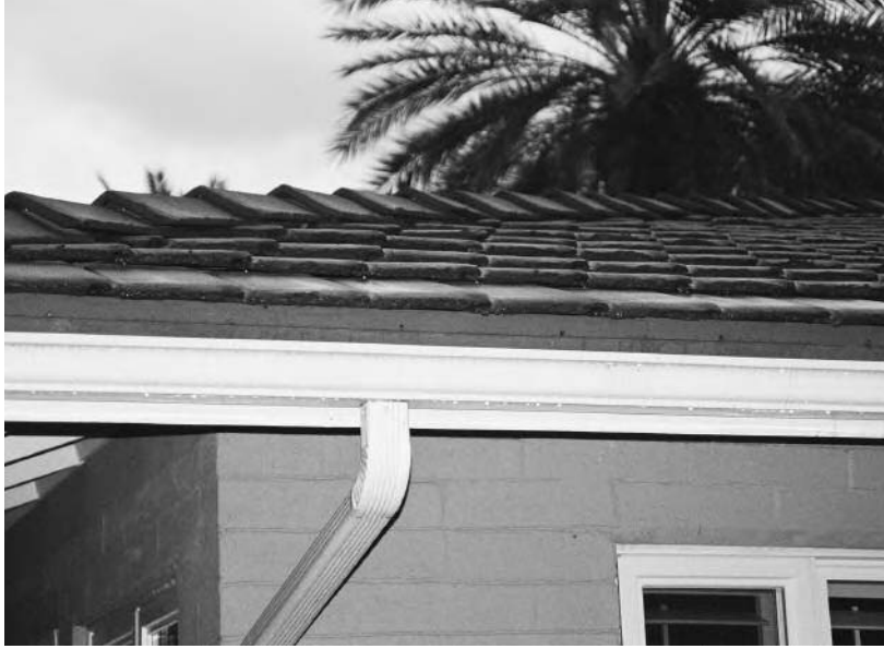
Downspout attached to a gutter
