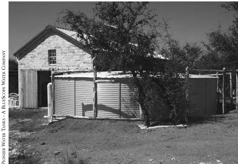
A private residential 35,000 gallon Pioneer Galaxy water storage tank used for rainwater collection in the hill country of Texas
