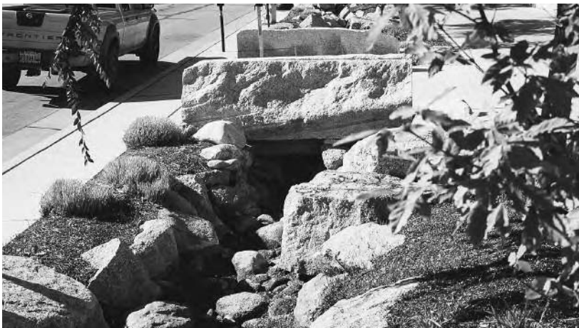
Passive rainwater harvesting: drainage swale next to sidewalk
