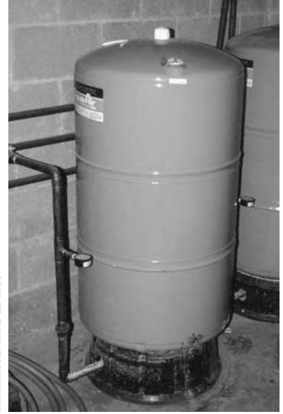
ABOVE LEFT: Multisiphon overflow unit with floating ball to eliminate backflow of fluids and smells and the stainless steel grill prevents rodents from entering the tank ABOVE RIGHT: Residential pressure tanks supply pumped rainwater from the cistern to clothes washing machine and toilets
