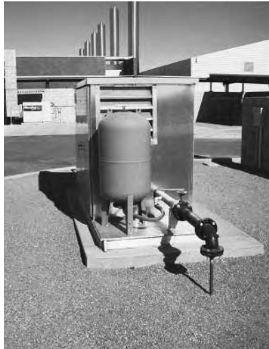
LEFT: Passive rainwater harvesting: Channel with drains to the landscape RIGHT: Pressure tank and equipment box
