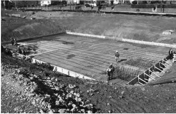
TOP LEFT: Cistern floor during construction TOP RIGHT: Cistern walls going up
