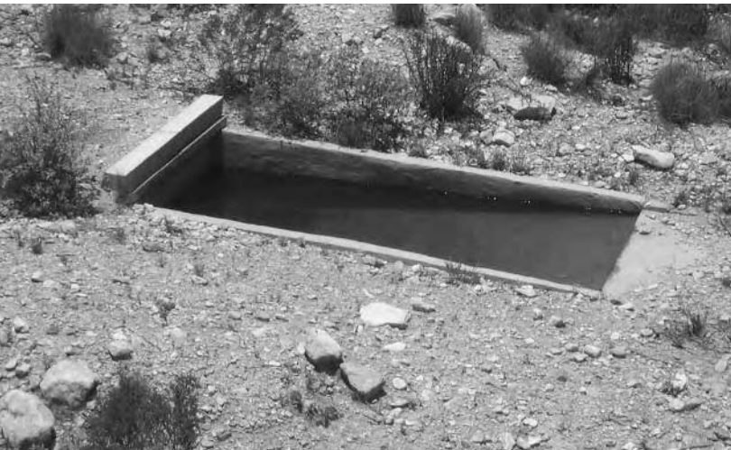
Concrete catchment trough for wildlife drinking
