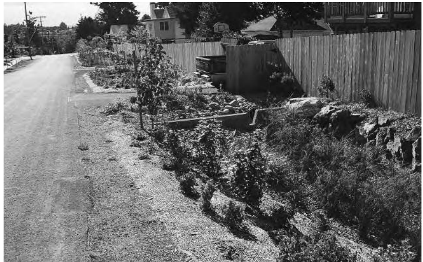
Younger rain garden where vegetation has not reach maturity; this is a cascade garden
