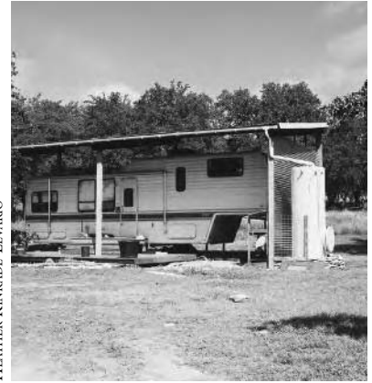
Mobile trailer under a rainbarn that is attached to a cistern
