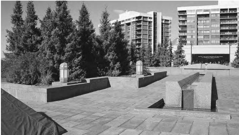
Passive rainwater harvesting: green roof on church in Salt Lake, UT
