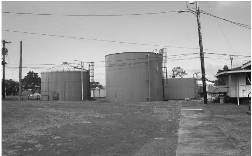
Water storage tanks
