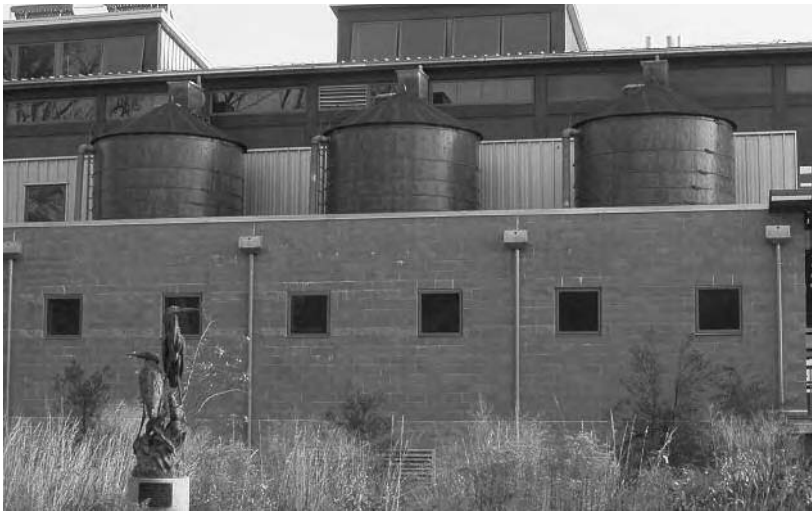
Close up of the pickle barrels used for cisterns
