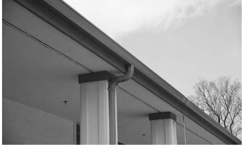
View of gutters and downspout connection
