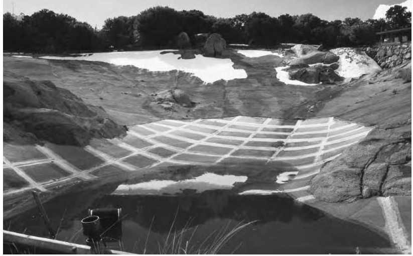
Upper catch basin
