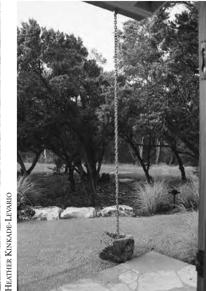
LEFT: Rainchain at spa RIGHT: Rainchain from extended gutter at spa
