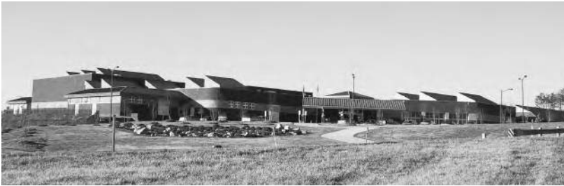
View with drop-off area at center
