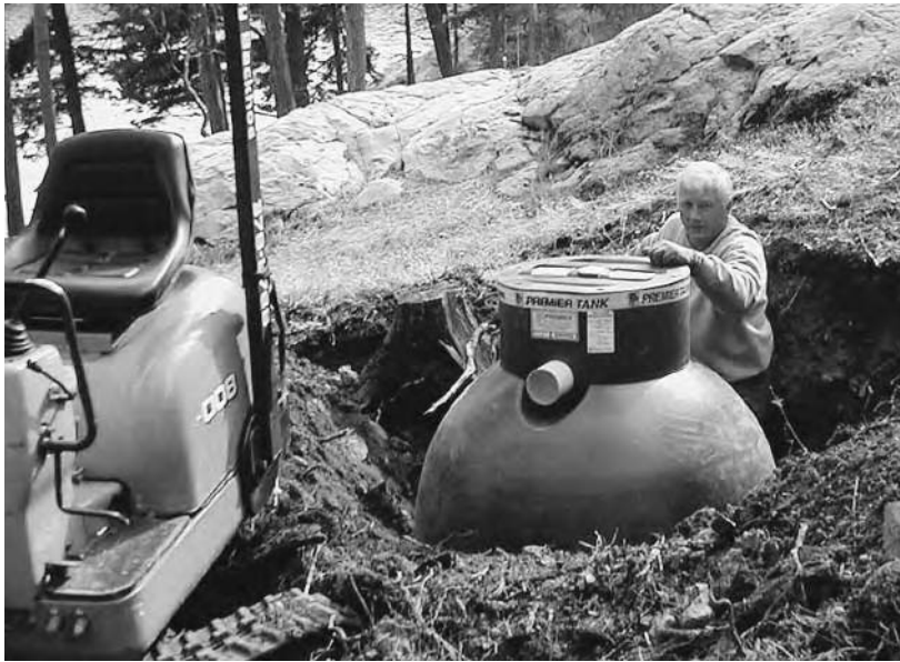
A 240-gallon collection tank from which collected rainwater is pumped to a remote storage tank
