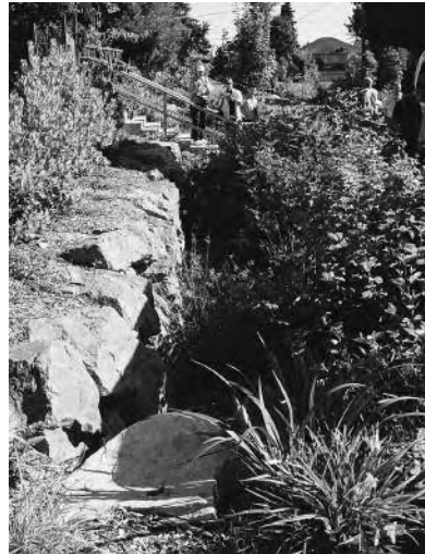
LEFT: Drain pipe emptying into a rain garden RIGHT: Rain garden between two drives; this is a rain garden running with the contours of the land
