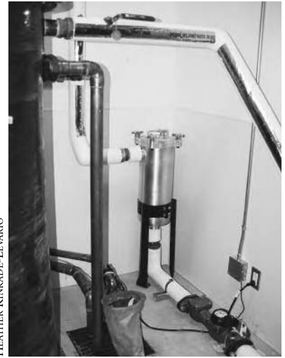
Bag filter and used filter to the side
