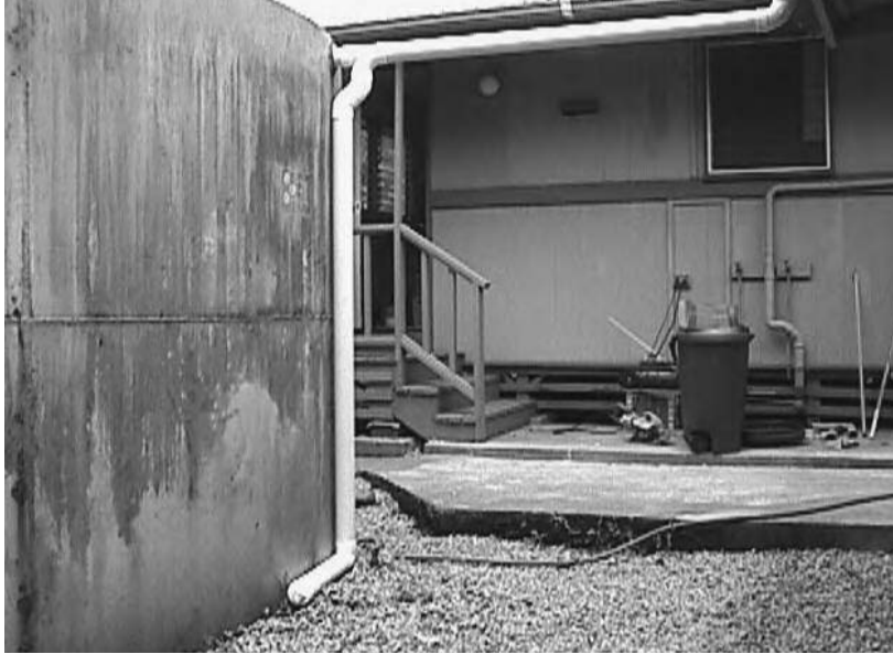
First-flush on a Hawaiian rainwater tank
