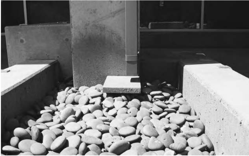
Downspout to rock splash pad
