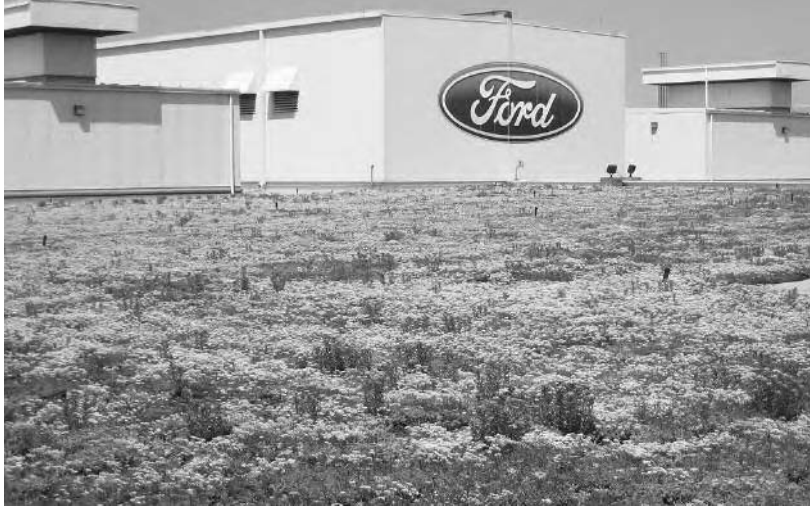
TOP: Green roof over assembly building LEFT: Rouge Visitor Center rainwater tank, inside the building for display. BOTTOM LEFT: Porous parking lot after completion in 2003 BOTTOM RIGHT: Ford Motor Company Visitor Center rainwater tank schematic
