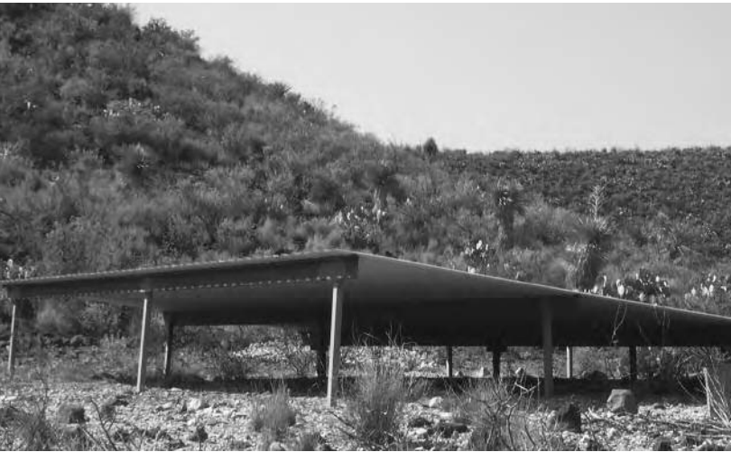
Raised "roof-like" catchment surface
