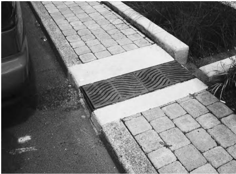
Green Streets Project: inlet with asphalt diversion dam
