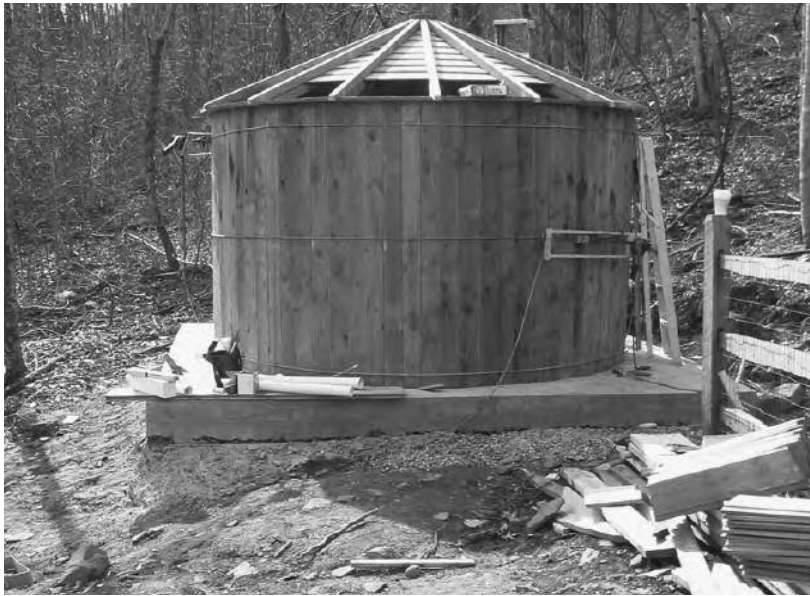
Wooden tank construction in cold climate – roof
