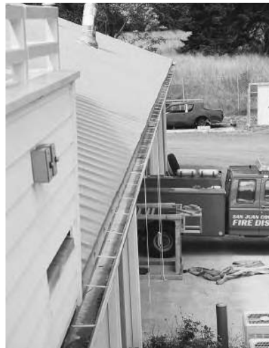
View of gutters from above
