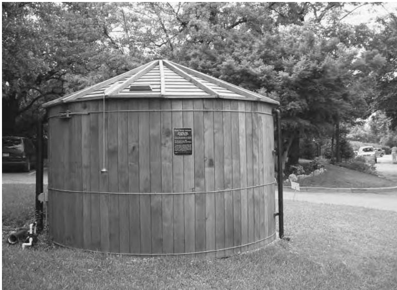
Fort Worth Botanical Gardens which has a 5,000-gallon TimberTank for irrigation of plants
