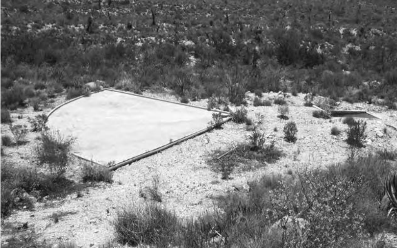
Concrete catchment pad for collecting water
