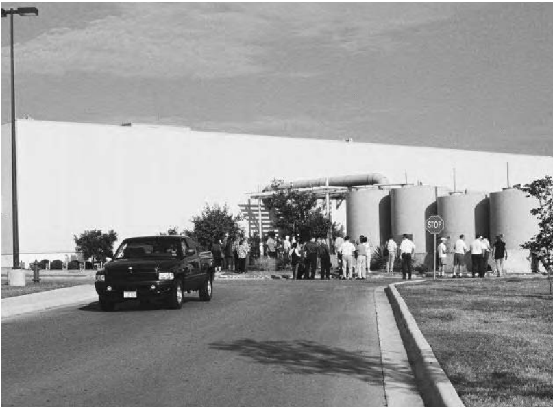
HEB store displays rainwater tanks at their entry road, Austin, TX
