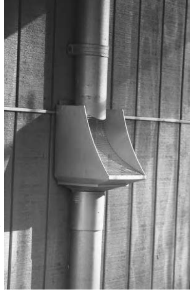
LEFT: Leaf Eater downspout filter (or rainhead) mounted in the traditional way at the gutter.
