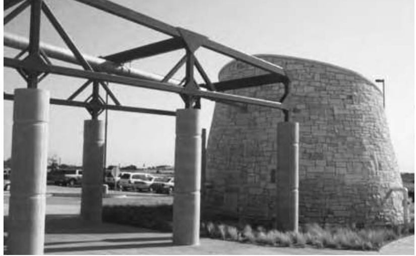
Gutter connection through a pipe to the front cistern
