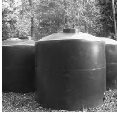
A 2,000-liter residential rainwater tank with a stand pipe and leaf catcher RIGHT (TOP TO BOTTOM): Private residential Pioneer Galaxy water storage tank in Western Australia Three black poly water storage tanks, 2,340 gallons each
