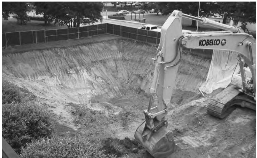
Excavation for the rainwater tanks next to the Legislative Building
