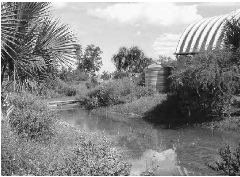
World Birding Center: A tank next to the arched roof catchment that feeds the adjacent wildlife pond
