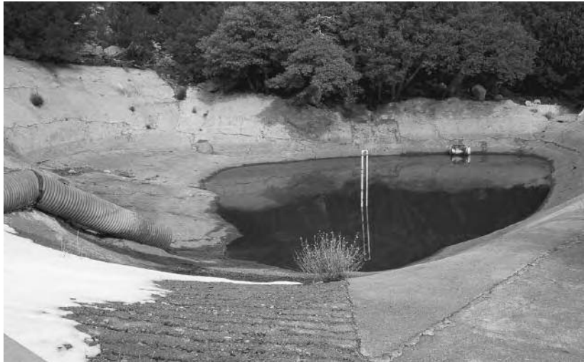
Lower catch basin
