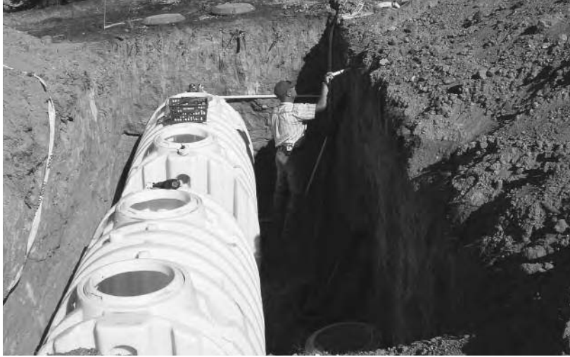
Dual cisterns being connected to drainpipes
