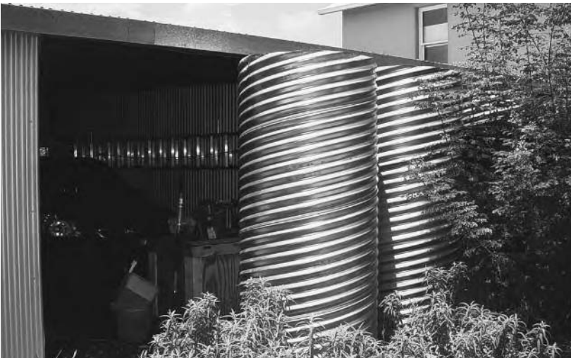
Two tanks in adjacent courtyard at the end of the carport
