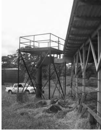
LEFT: Catchment surface collection pipe RIGHT: Flume from catch- ment surface to storage tank
