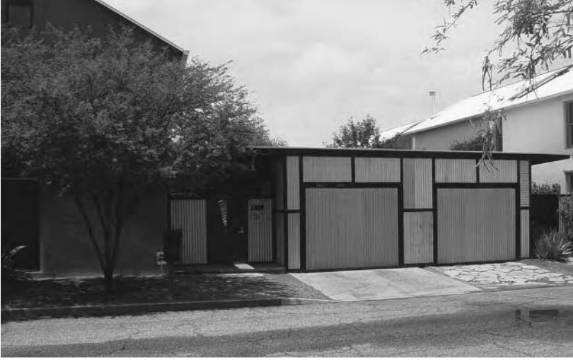
View of the four-home quadplex and carports from the street after carport completion
