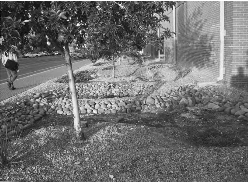
University of Arizona, Tucson, Arizona stepped stormwater basins adjacent to a building, note gutter down- spouts feed each basin
