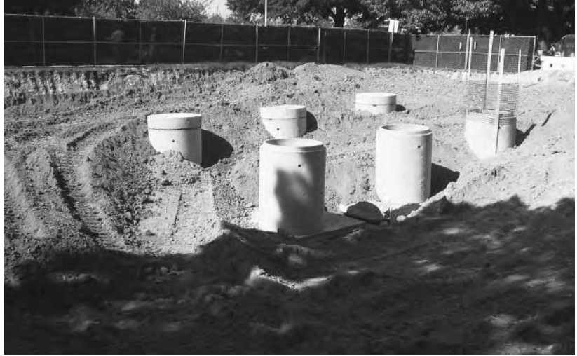
Exposed manholes and covered tanks
