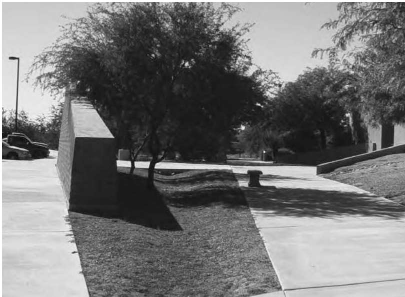
Passive rainwater harvesting: Pima Community College swale next to sidewalk collects storm-water runoff for vegetation
