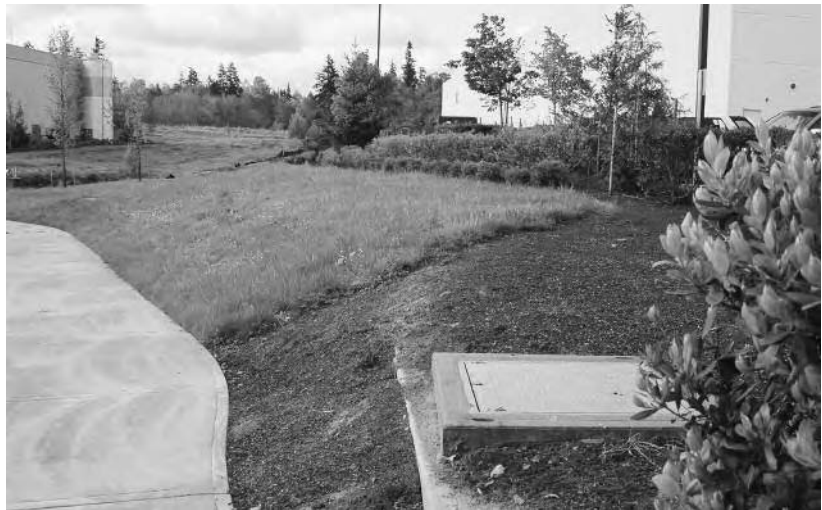
Landscape on east end of the building, where the rainwater tank is buried and tank access hatch is located
