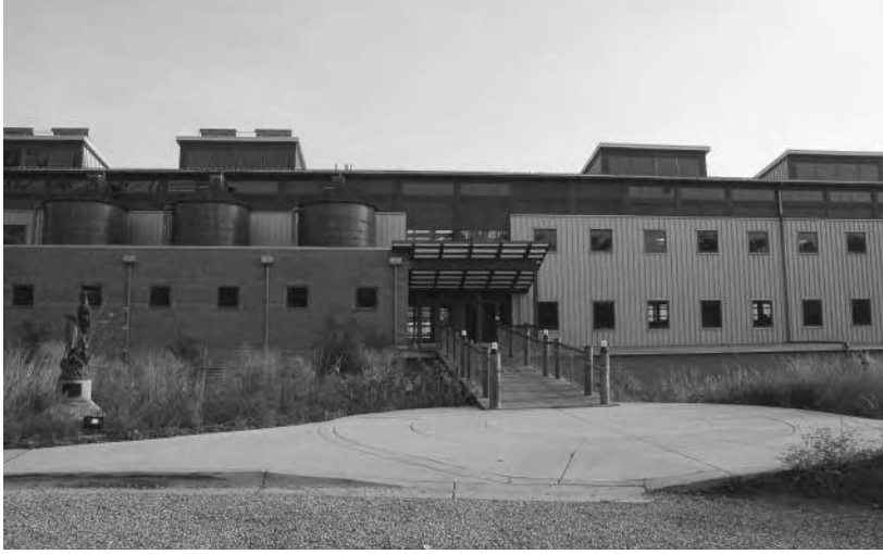
Front of building, with cisterns
