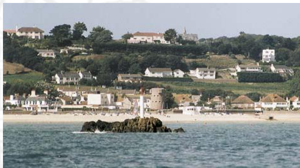
Sillette Passage Leading Marks in line 000° (8.39.3)
