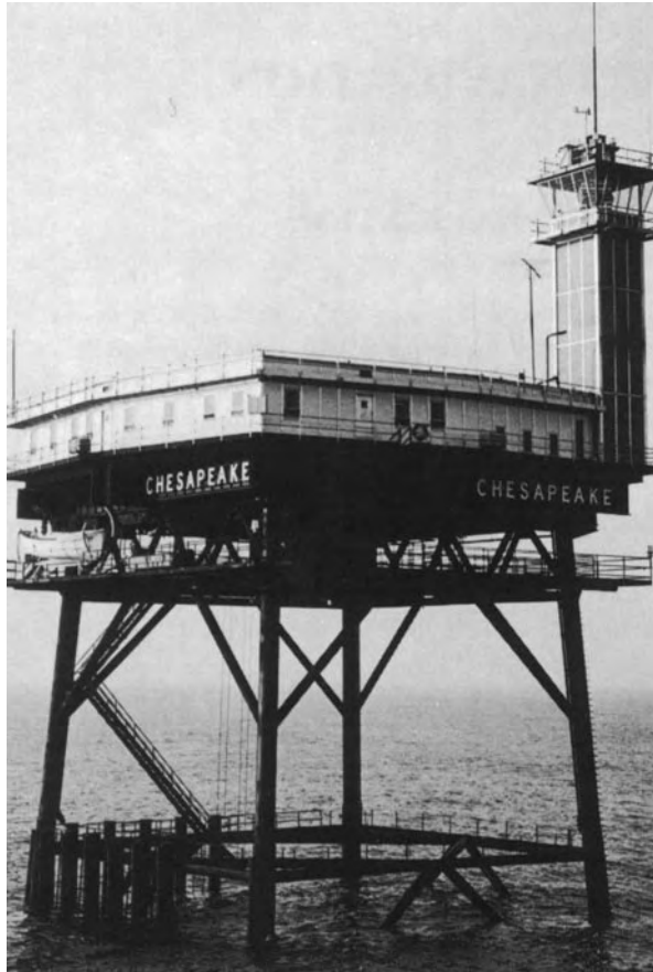
Figure 501a. Typical offshore light station.
