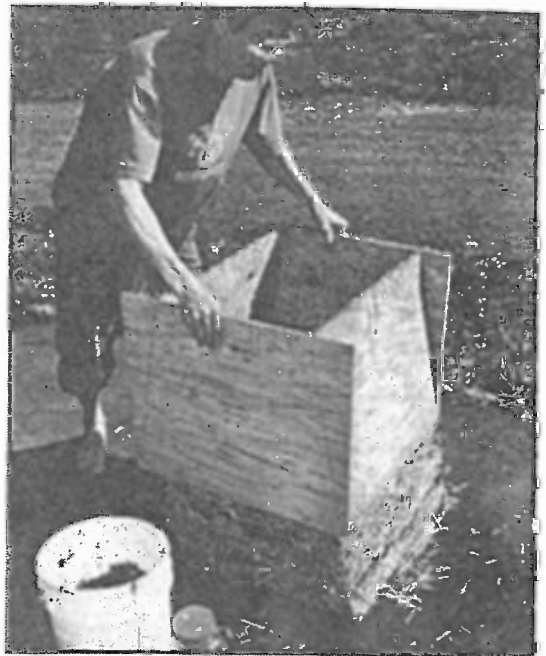
Figure 305. After 4-6 layers, the frame is lifted off, and the process begins anew.
