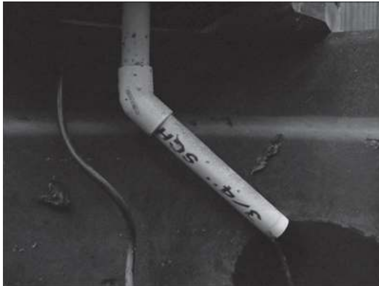
A Coanda drain beneath a grow bed. The 45-degree angle aids in forming a hydrodynamic plug to start the siphoning action for a bell siphon or internal loop siphon. The dust is an indication of how long it's worked without needing adjustment.
