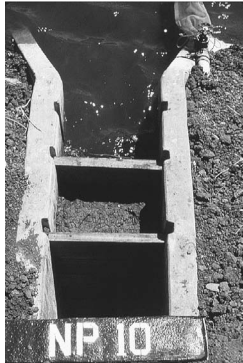
Figure 8. A simple kettle design has two sets of boards set in slots to control the water level. Dirt is packed between the two sets of boards to deter leakage. Valves are not required in conjunction with this type of kettle, but a good deal of labor is needed to put the dirt in place and then remove it. The third pair of slots show the location of the screen.
