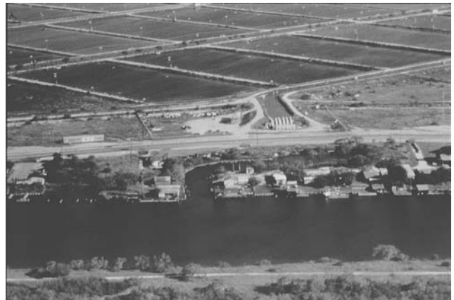
Figure 16. Aerial photo of intake at Arroyo Aquaculture Association farm in Texas. (Photo by Louis Hamper.)
