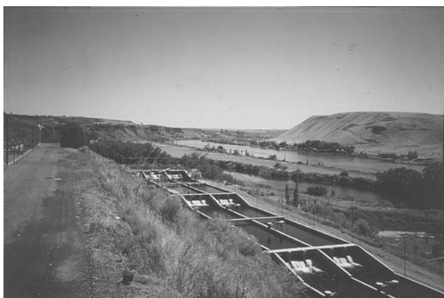
Figure 6. Outdoor raceways. Note the demand feeders.
