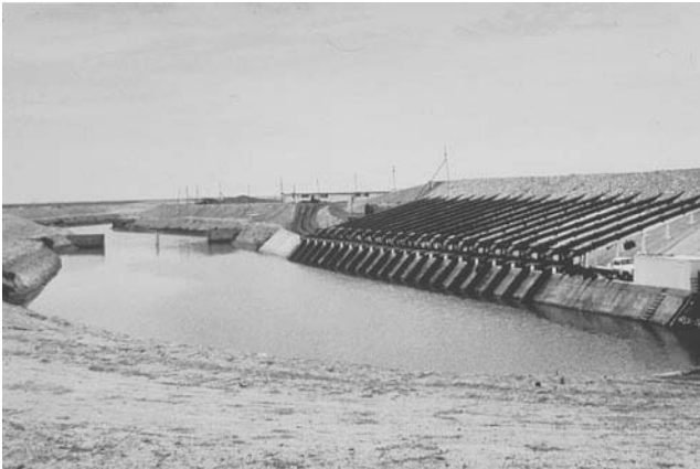
Figure 33. Large shrimp farm intake and reservoir in the Salinas, Ecuador.
