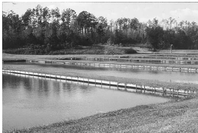
Figure 3. Ponds with vertical sides constructed of wood. This approach allows for the construction of narrow between pond levees, but will add to the cost of construction.
