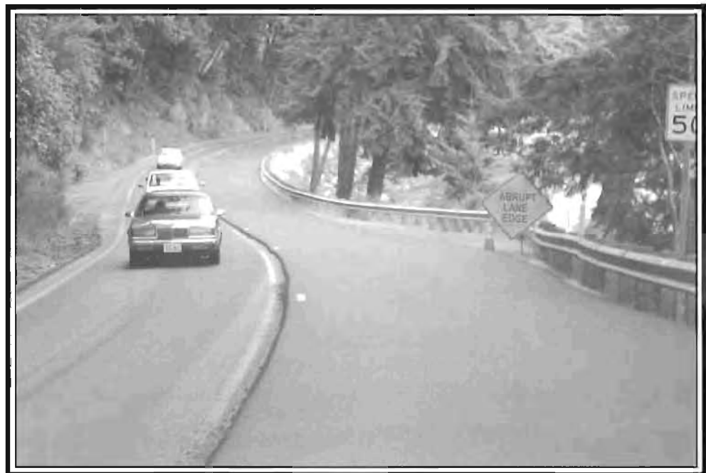
You can usually translate this sign to mean Watch for Edge Traps.
