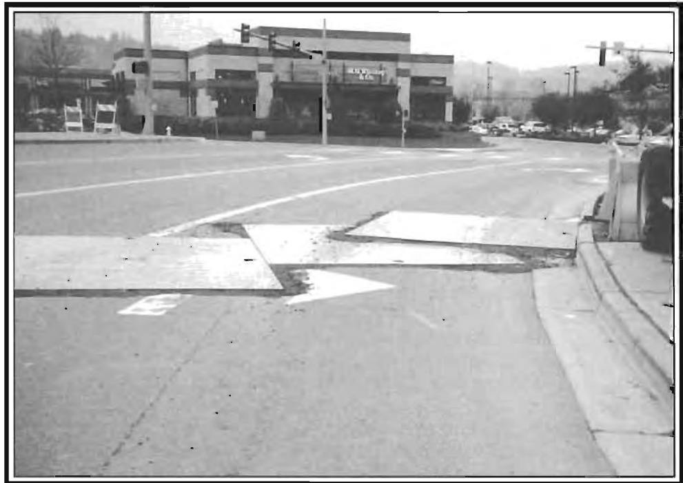
When crossing slippery steel construction plates, get the bike vertical, stabilize speed, and pick a path that avoids the sharp edges.
