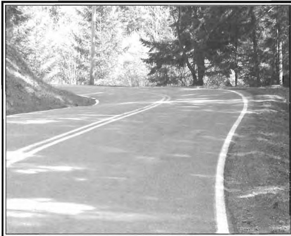
If the opposite edge disappears, that's a hint the pavement slants the wrong way (off-camber)
