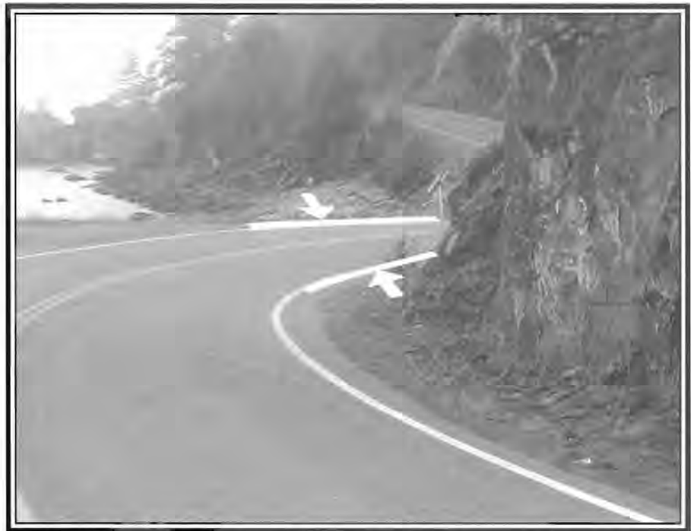
If the opposite edge of the pavement appears to be getting closer to the inside edge (converging), then the corner is either tightening up or off-camber.
