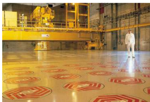
■ Figure 29 The EEV-SE facility for the interim storage of vitrified HL waste
