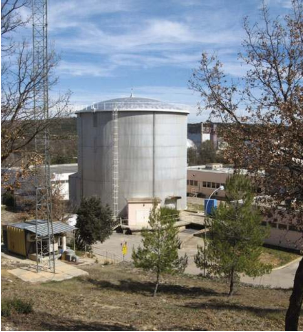
■ Figure 40 View of MASURCA reactor containment
