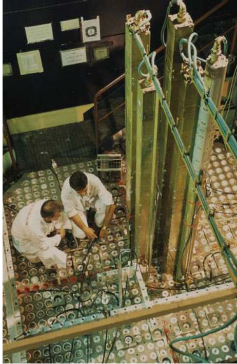
Figure 44 View of suspension table and safety rods mechanisms
