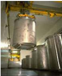
Claddings enrobed in concrete
