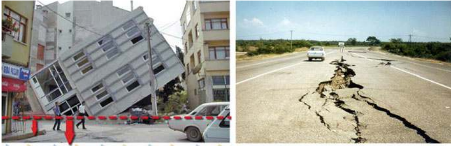
Figure 184 Physical damages of earthquakes
