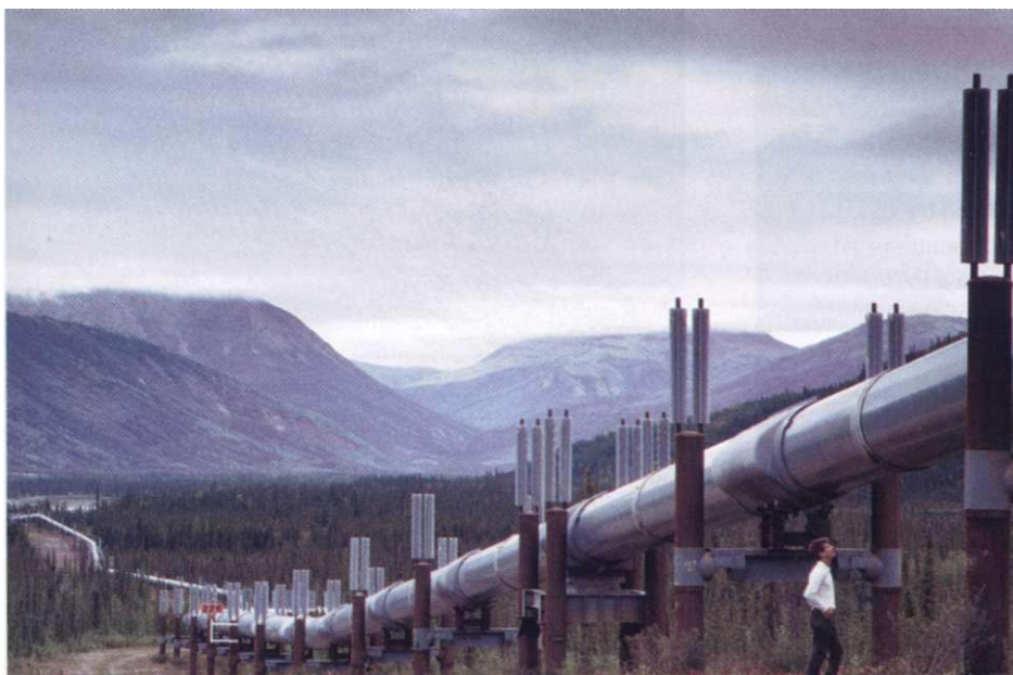
Figure 21.20 Along its 1300-km route from Prudhoe Bay to Valdez, the Alaska oil pipeline crosses 675 km of permafrost, perched on specially designed vertical supports. Because thawing of the permafrost would cause the supports to become unstable, they are outfitted with heat pumps designed to keep the ground around them frozen. The heat pumps contain anhydrous ammonia that vaporizes below ground and rises and condenses above ground, discharging heat through the two aluminum radiators atop each of the vertical supports. [Galen Rowell/Corbis.]
