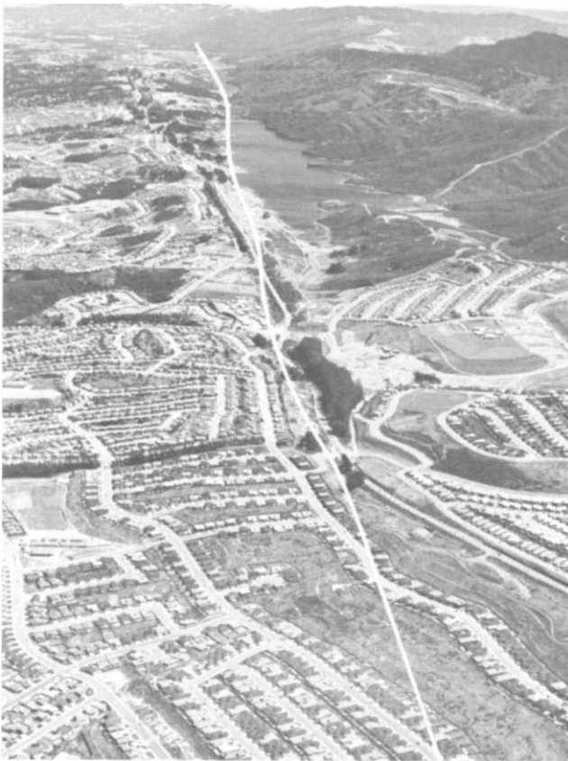
Figure 13.21 Housing tracts constructed within the San Andreas fault zone, San Francisco Peninsula, before the state passed legislation restricting this practice. The white line indicates the approximate fault trace, along which the ground ruptured and slipped about 2 m during the earthquake of 1906. [R. E. Wallace/USGS.]
