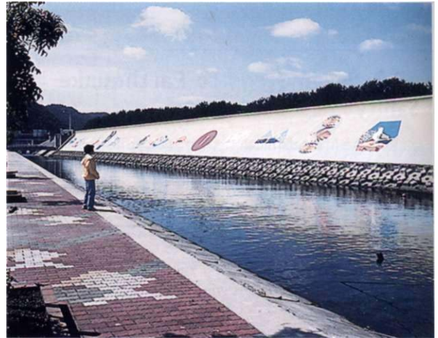
Figure 13.22 Tsunami barrier in the town of Taro, Japan. [Courtesy of Taro, Japan.]
