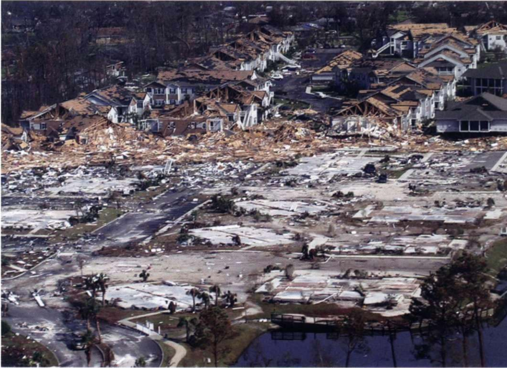
Figure 20.7 Hurricane storm surge along coastlines may result in the complete destruction of residential buildings, which pile up as lines of debris well inland of the normal coastline. The damage seen here was caused by Hurricane Katrina. [U.S. Navy/Getty Images.]
