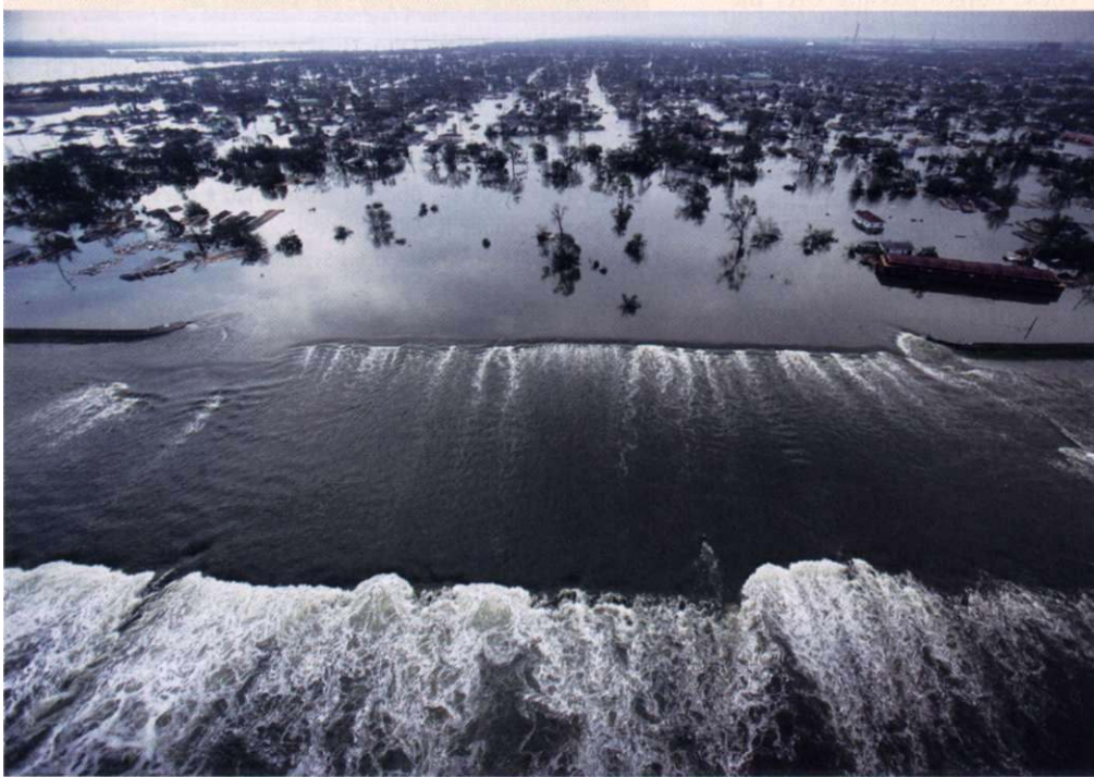
Water spills over a levee along the Inner Harbor Navigational Canal and floods the inner city of New Orleans. [Vincent Laforet-Pool/Getty Images.]
