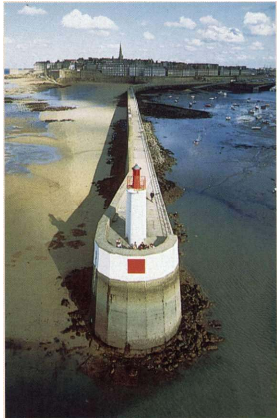
Construction of groins along a shore to control erosion of a beach may result in erosion downcurrent of the groin and loss of parts of the beach (right of groin) while sand piles up on the other side (left of groin). Longshore current flows from left to right. [Philip Plisson/Explorer.]
