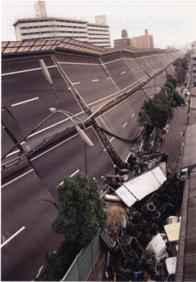
Figure 13.15 This elevated expressway, in Kobe, Japan, was overturned during an earthquake in 1995. [Tom Wagner/Corbis/SABA.]
