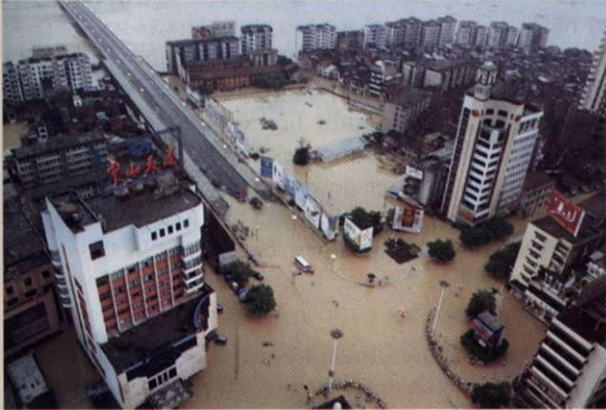
Like many cities built on river floodplains, Liuzhou, China, is subject to flooding. This flood, in July 1996, was the largest recorded in the city's 500-year history. [Xie Jiahua/China Features/Corbis Sygma.]
