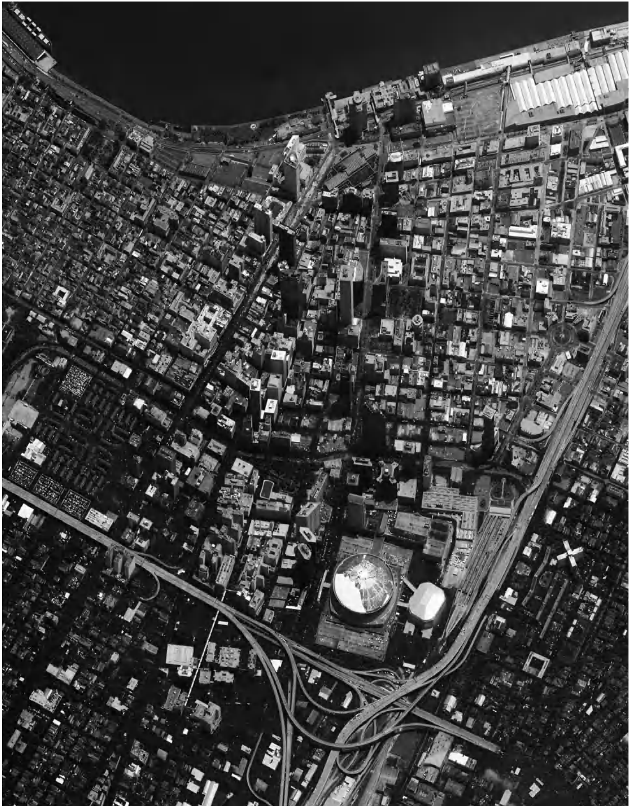
Fig. 8.8c,d Hurricane Katrina in 2005 has left severe damage in the Mississippi delta region, USA. The Louisiana Superdome was converted into an island refuge for as many as 30,000 people. Many sheltered in the stadium while Hurricane Katrina raged overhead on Monday, August 29, 2005, and many more have been brought to the Superdome after being rescued from their flooded homes. The stadium itself was surrounded by flood water when the Quick Bird satellite captured this detailed image on August 31. Much of the stadium's bright white roof is missing. (Photo credit: NASA).
