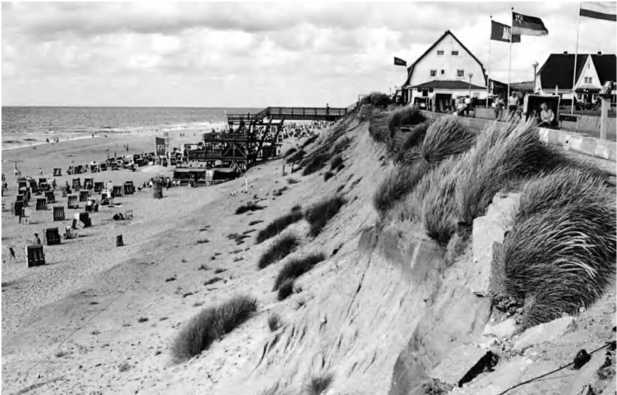
Fig. 4.51 Cliffs may also exist for a short time as quasi stable features in sand as in these mid-Holocene dunes with soil development and vegetation cover of Sylt Island, German North Sea coast. Many houses have been destroyed by rapid cliff retreat in these dunes during the last 200 years. (Photo credit: D. Kelletat).
