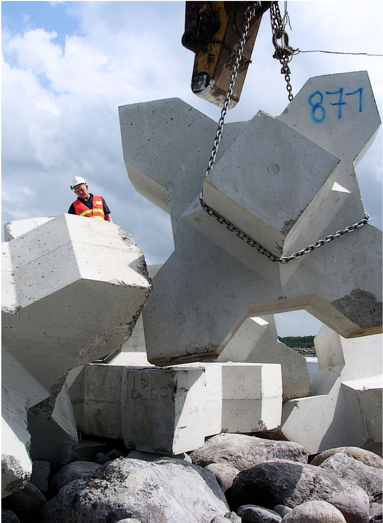
Fig. 8.37 a,b Coastal protection with tetrapods changes sandy beaches into concrete constructions to combat ongoing beach erosion and sea level rise. Sylt Island, German North Sea coast. (Photo credit: a) D. Kelletat; b) ©Van Oord).
