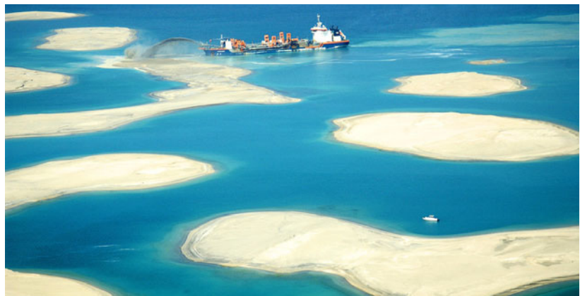
Fig. 8.41 c,d Artificial beach nourishment of The World, Dubai (Photo credit: ©Van Oord)
