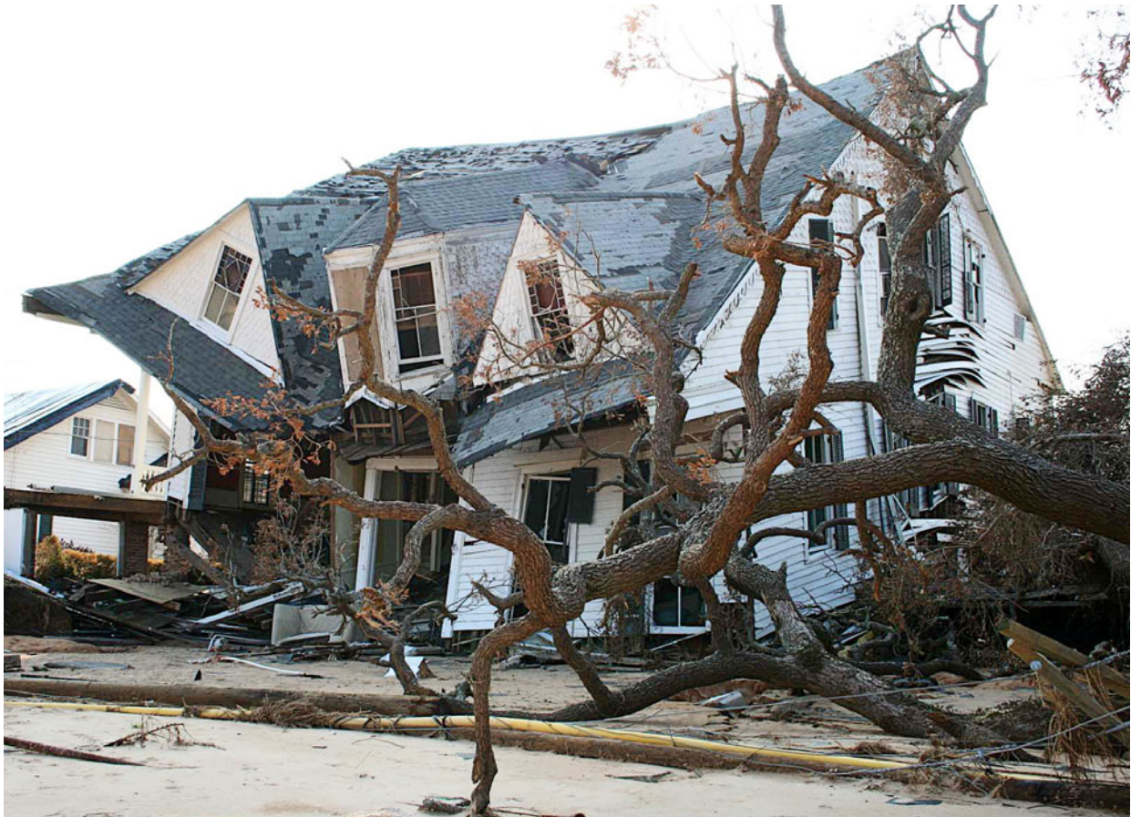
Fig. 8.8a,b The combined destructive forces of extreme wind velocities, record storm surge and up set waves from Hurricane Katrina (2005) left these signatures at single structures (a) and wiping out parts of settlements along the US Gulf coast near New Orleans (b) (Image credit: National Oceanic and Atmospheric Administration/Department of Commerce and National Coastal Data Development Center (NCDDC).
