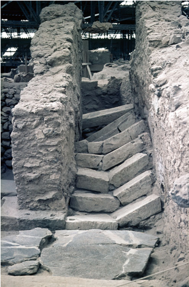
Fig. 1.8 (a) A staircase in the Minoan settlement (>3,500 years) of Akrotiri on the island of Santorini/Thira (Aegean Sea, Greece) has been destroyed by compression forces during an earthquake in early historical
