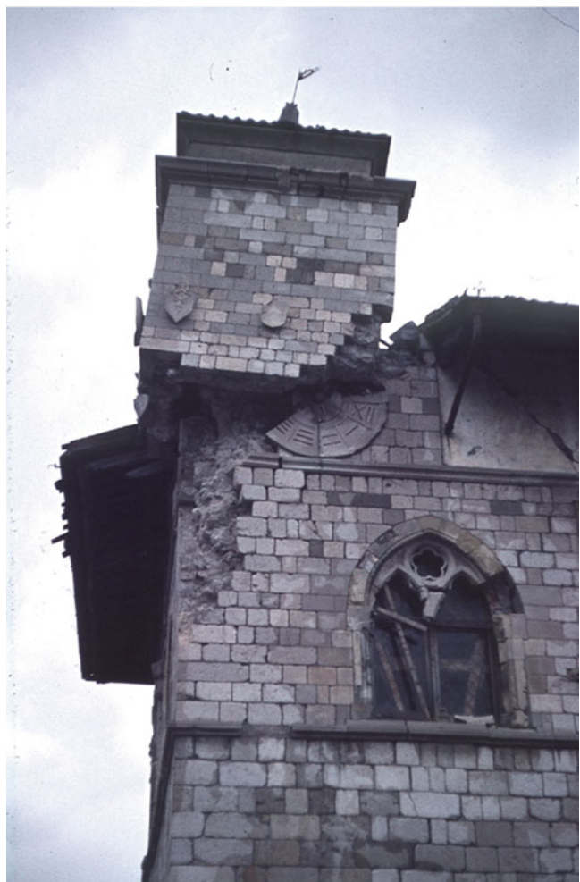
times. (b) Sideward displacement of the mayor's house in the medieval township of Venzone (northeast Italy) during an earthquake 50 years ago. The small roof tower stayed almost at its old place.
