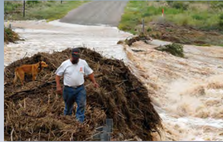
FIGURE 10-B A raging flash flood deposited this pile of debris and washed out a road near Hagerman, New Mexico, in July 2009. (AP Photo/Roswell Daily Record, Mark Wilson)
