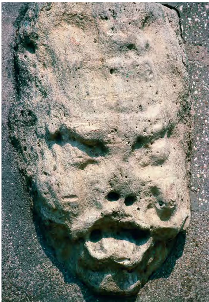
Figure 13-21 Acid rain accelerates the chemical weathering of stone monuments and structures. (Photo by Adam Hart-Davis/Science Photo Library/Photo Researchers, Inc.)
