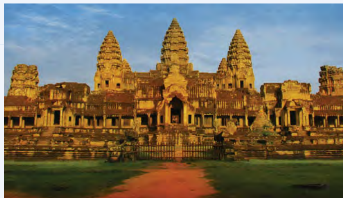
FIGURE 15-C This ancient temple at Angkor Wat, Cambodia, was built of bricks made of laterite. (Photo by Nestor Noci/Shutterstock)
