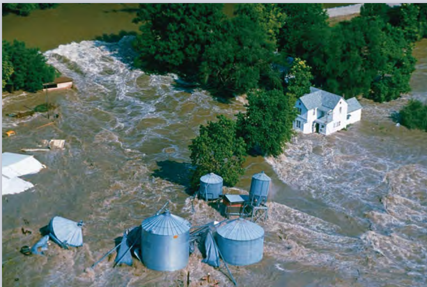
FIGURE 9-C Water rushes through a break in an artificial levee in Monroe County, Illinois, in 1993. During the record-breaking floods of 2008 and 1993, many levees could not withstand the force of the floodwaters. Sections of many weakened structures were overtopped or simply collapsed. (Photo by James A. Finley/AP/Wide World Photos)
