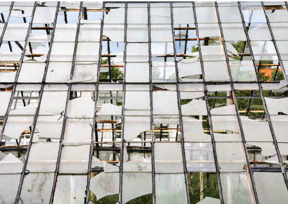
Figure 5-22 Hailstorm damage to a greenhouse. (Photo by McPHOTO/KPA/agefotostock)
