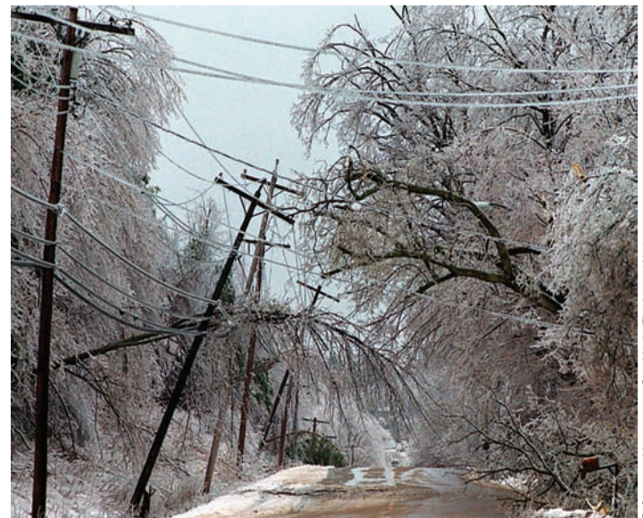
● FIGURE 1.20 An ice storm near Oswego, New York, in January 1998 caused utility poles and power lines to be weighed down, forcing road closure.
