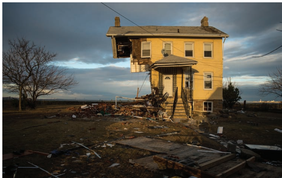
● FIGURE 16.31 A home destroyed by Hurricane Sandy in Union Beach, New Jersey. Sandy devastated parts of coastal New Jersey and New York, causing more than $50 billion in damages.
