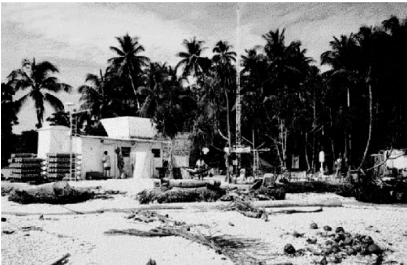
Figure 21 NCAR ISS in Kapingamarangi, Pohnpei State, Federated States of Micronesia. A wind profiler antenna is pointed vertically and shrouded by a clutter fence visible on top of the shelter. Aluminum cylinders shield a portion of a RASS radio acoustic sounding system. See ftp site for color image.
