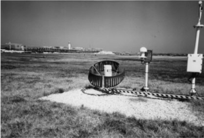
Figure 24 Sensors located too close to a jet takeoff area. Windscreen around the rain gauge is damaged from jet blast. Blast also causes temperature to rise and wind gusts to increase. See ftp site for color image.
