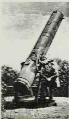
Figure 2.29 (Right) Refinement of Nasmyth's idea gives basis of modern coudé system.
