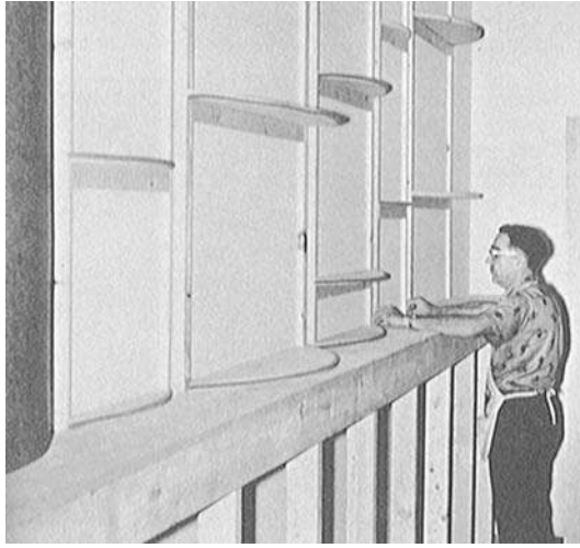
FIGURE 12-27 The construction of polys in a motion picture sound mixing studio. Foam rubber anti-rattle strips are applied on the edge of each bulkhead. Also note the random spacing of the bulkheads. ( Moody Institute of Science )
