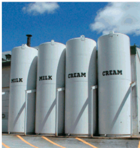
This ice cream plant in Burlington, Vermont, uses cylindrical containers for its milk and cream.
