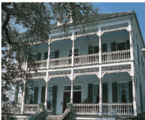
In a hot climate, a deep overhang shelters windows from the sun.
