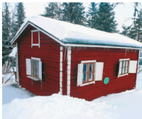
In a cold climate, a narrow overhang lets in more light and warmth.
