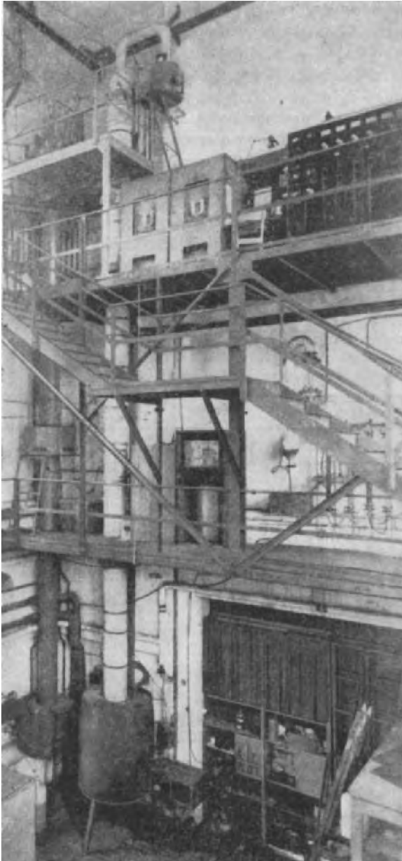
Fig. 160 The author's still for enriching \text{H}_2^{18}\text{O}
