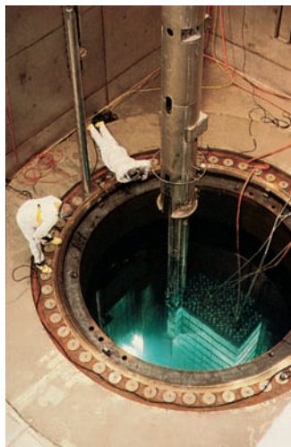
Figure 21.11 Refueling the core of a nuclear reactor.
