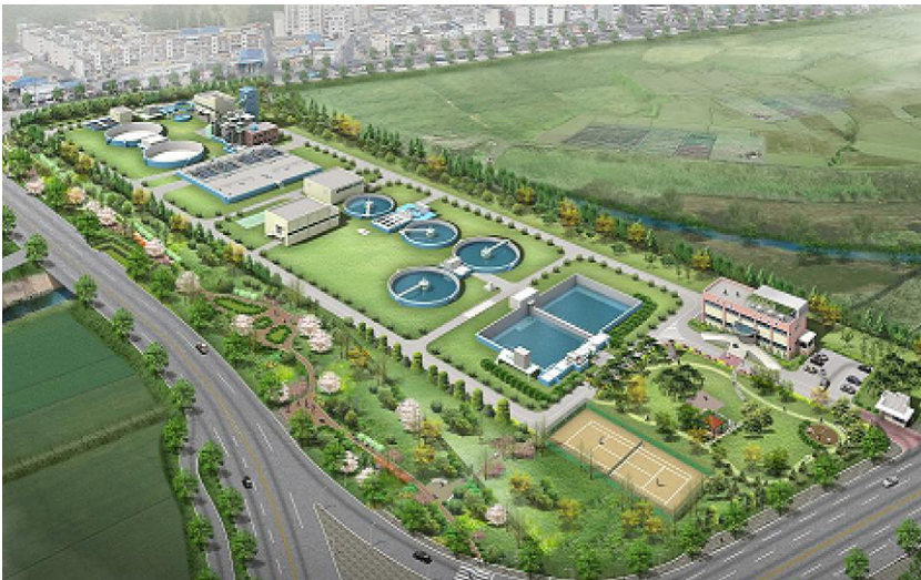
FIG. 5.44 The Dalsung WwTW site.
