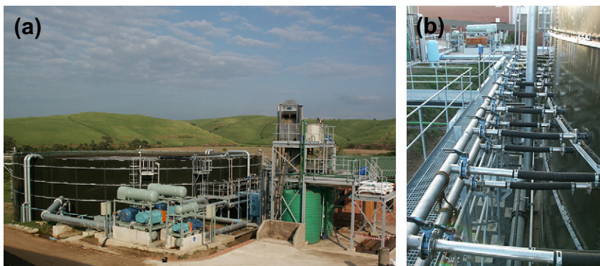
FIG. 5.11 The Illovo Sugar plant: (a) the biotank and (b) connections from the upper and lower decks of the membrane units in the biotank.
