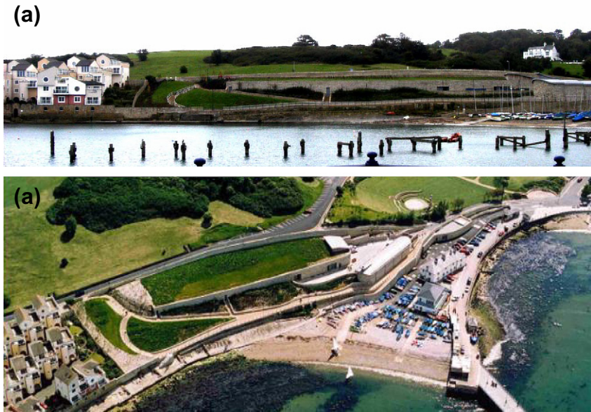
FIG. 5.4 View of Swanage sewage treatment works: (a) from the sea and (b) from the air.
