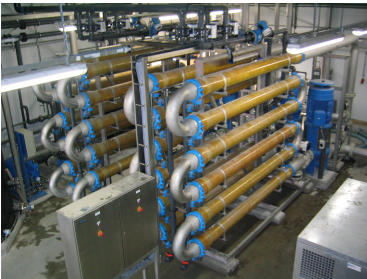
FIG. 5.51 The sidestream MT modules at Eemshaven.
