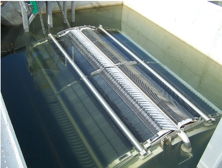
FIG. 5.18 The Huber VRM unit being installed at Arenas de Iguña.
