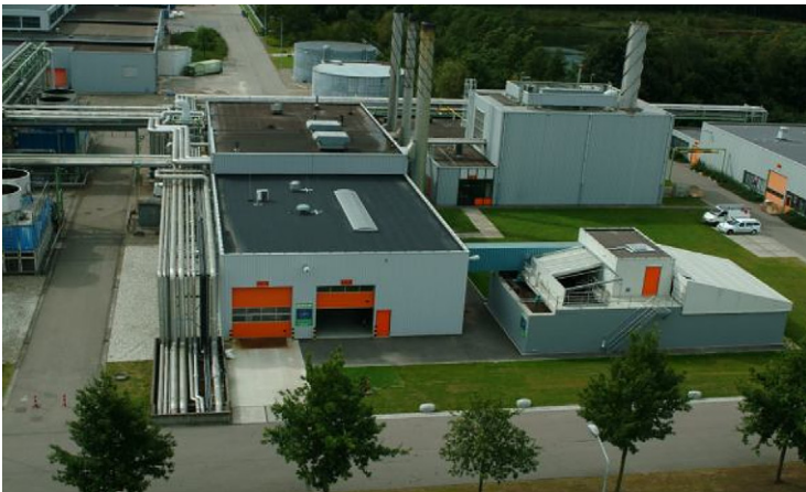
FIG. 5.22 Overview of plant at Tilburg. Front right: MBR plant building; front left: building housing RO, dewatering unit, storage of chemicals and permeate and control room.
