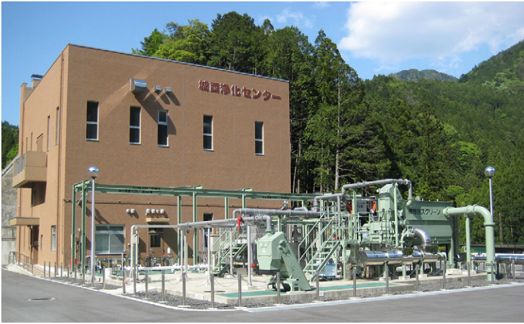
FIG. 5.40 The MBR plant at Hamamatsu City.
