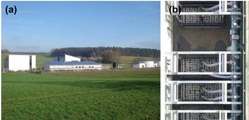
FIG. 5.47 The MBR plant at Monheim: (a) the site and (b) plan view of the membrane modules.
