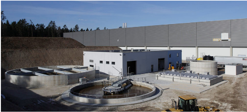
FIG. 5.19 The WwTW at Hans Kupfer & Sohn.
