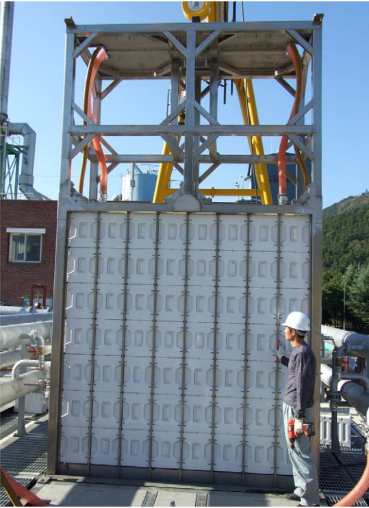
FIG. 5.45 A single 112-cartridge frame being installed at Dalsung.
