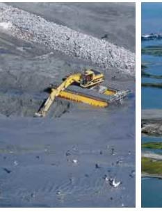
and water at the feet of the land crew. The men on the island let the water drain off and the sediment accumulate. The quantity of runoff is carefully calculated to ensure that enough sand builds up. The engineers have estimated a cut-to-fill ratio of 1.5 for this project; in other words, about a third of what is taken from the Gulf floor washes away when it reaches the island. By the end of the project, nearly three million cubic yards of watery sand will have been pumped into East Timbalier.
