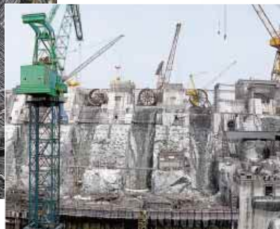
FEEDING THE TURBINES: Huge water intakes ( left ) will divert water from the Yangtze River to one of 26 gigantic turbines. At full capacity the dam will generate 18,200 megawatts, making it the biggest hydropower producer in the world. The intakes are placed about halfway up the dam's eventual 60-story height ( below ).
