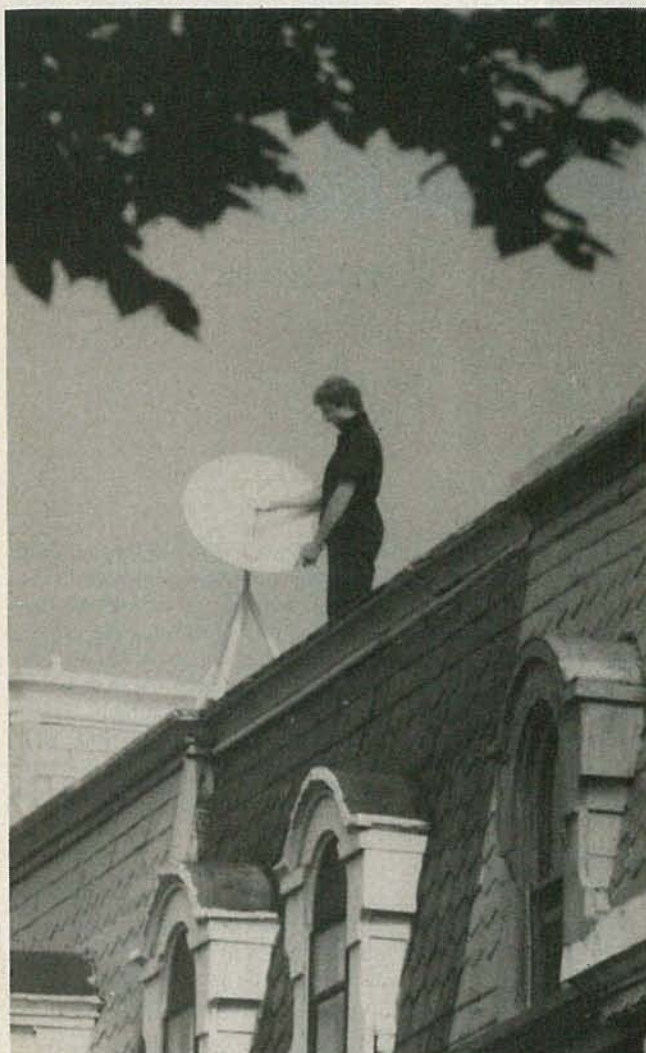
THE MAIN ADVANTAGE OF DBS is that smaller dishes can be used because of the high power of the satellite transponders. That means that you can receive DBS programming even in a city.
