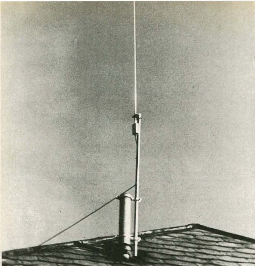
An active-antenna system presents few mounting-problems.
