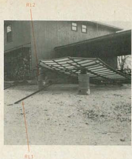
FIG. 21—THE TOP END OF THE ANTENNA is raised three to four feet off the ground so rear legs RL1 and RL2 can be attached. Put small blocks under the lower end to protect the corner adjustment bolts.
