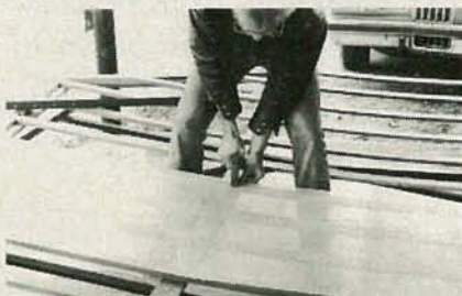
FIG. 15—KEEP TENSION ON THE SCREEN as you place the staples until you have tacked all around the edges. When working with the first strip of mesh you will have to stand between slats in the lattice.
