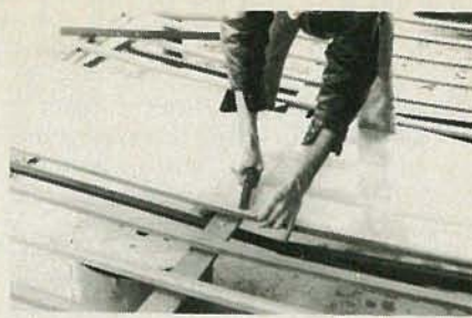
FIG. 16—AFTER STAPLING ONE EDGE, keep the screen taut and staple the point directly across from the first.
