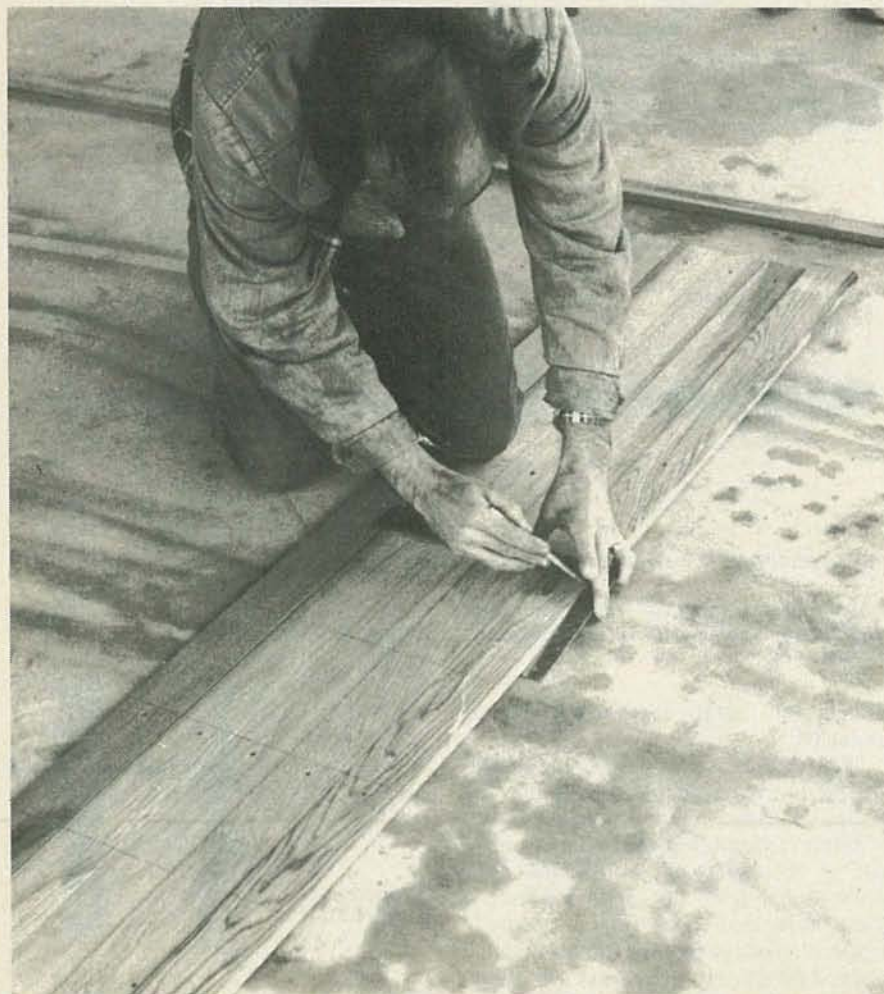
FIG. 8—MARK ALL FIVE VERTICAL STRIPS every eight inches to make installing the horizontal strips easier.
